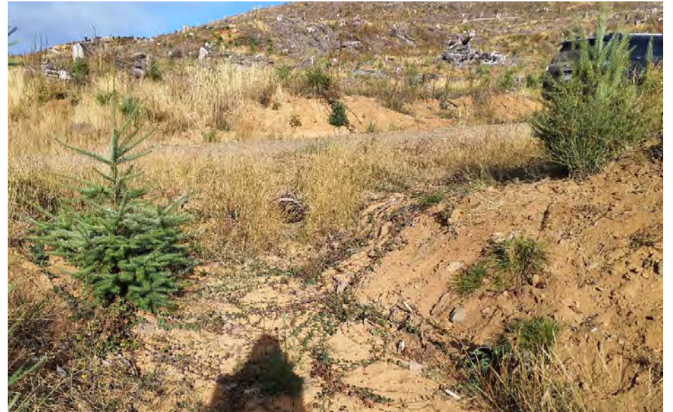
Photo 129. Culvert outflow is short, wide, and mostly unvegetated.. Looking NW. Taken: 10/11/2022. Lat/Long: 46.05114293, -123.2856082.
