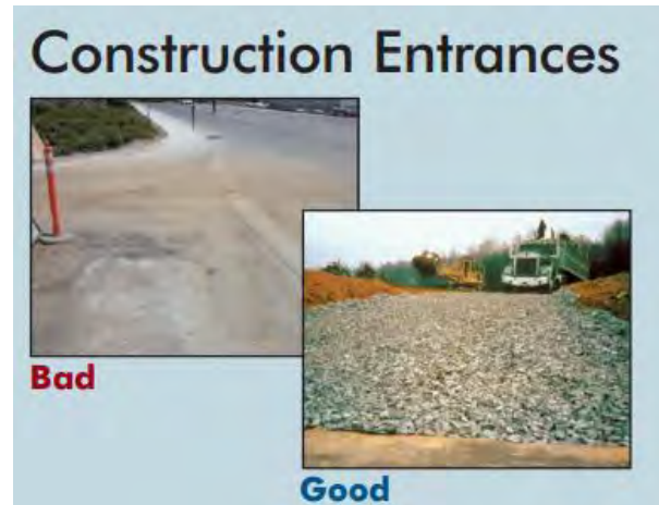
Figure 102. Stabilized gravel construction entrance examples (EPA 2003).
