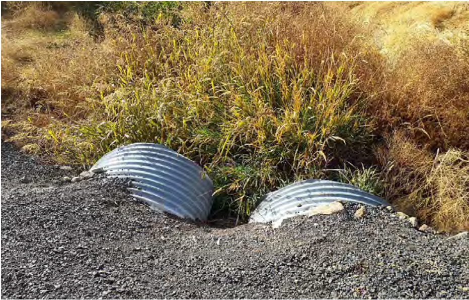
Photo 178. Double culvert under road drains riverine wetland to drainage on other side. Looking W. Taken: 10/22/2022.
