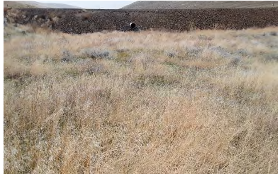
Photo 402. Culvert is perched coming out from under Butter Creek Rd, there is no bed or banks on this downhill end either. Looking NW. Taken: 11/14/2022.
