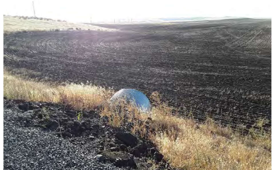
Photo 217. Culvert under road but no bed or banks in crop field or other evidence of flow. Looking NW. Taken: 10/23/2022.
