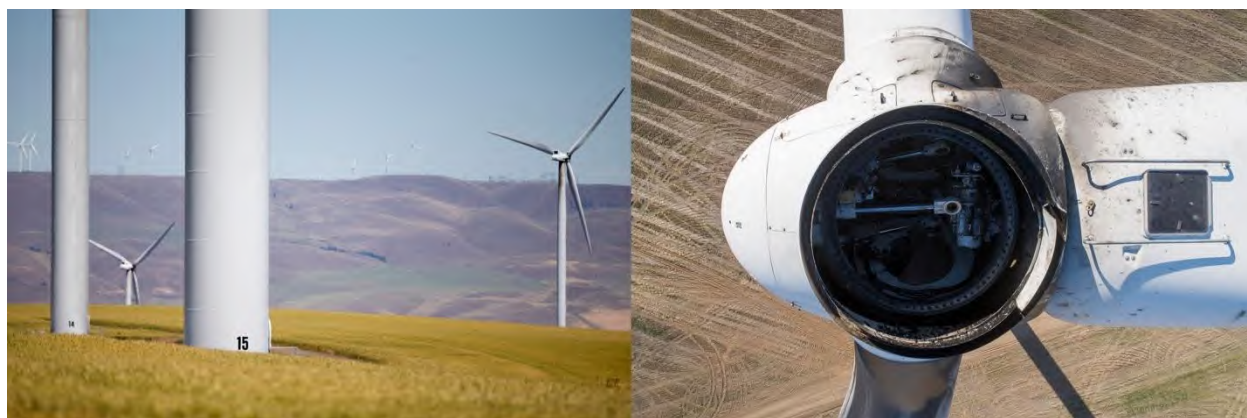
Farmers cultivate wheat right up to the base of wind turbines at Portland General Electric's Biglow Canyon wind farm (left). An aerial shot (right) of a Vestas turbine on Feb. 22, after it threw a blade 100 yards into a field below.
