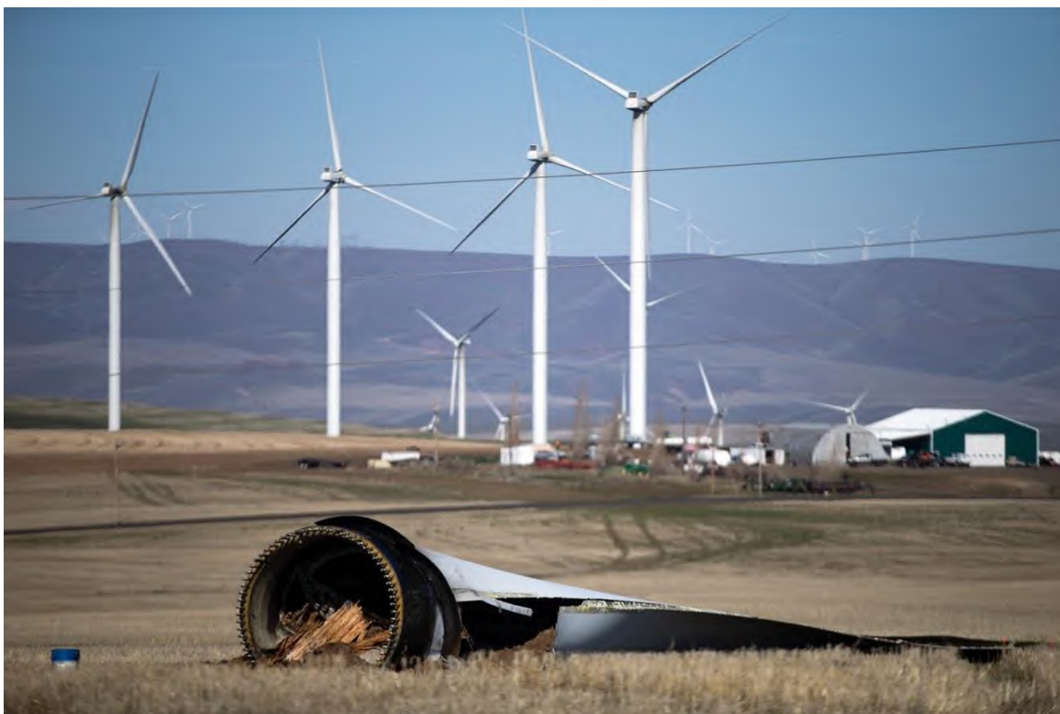
The blade thrown from a turbine at PGE's Biglow Canyon wind farm on Feb 1. An outbuilding next to the McCullough's residence is shown in the background.
