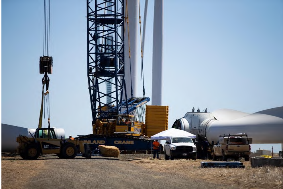
Workers replacing the blades on a Vestas V82 wind turbine at Portland General Electric's Biglow Canyon wind farm in late June. The turbine threw one of its blades into a wheat field on Feb. 1. PGE blamed "a loss of clamping force."
