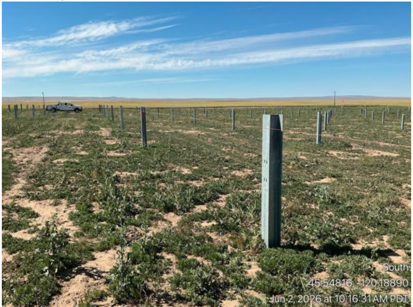
Photo 1. Solar panel foundation installation.
