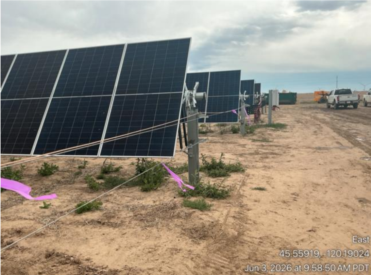
Photo 2. Solar panels are installed on foundations and trackers.
