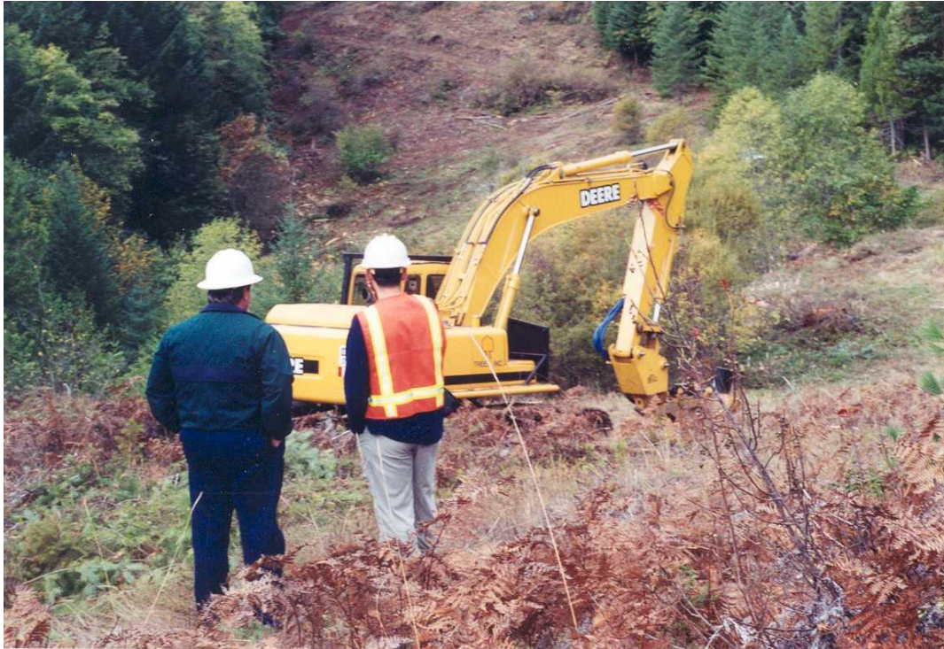
Figure 6.3. Right-of-way reclamation using mechanical control. In this case, a slashbuster.
