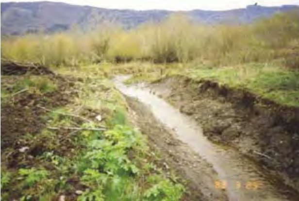
A newly excavated drainage ditch creates a drier water regime.
