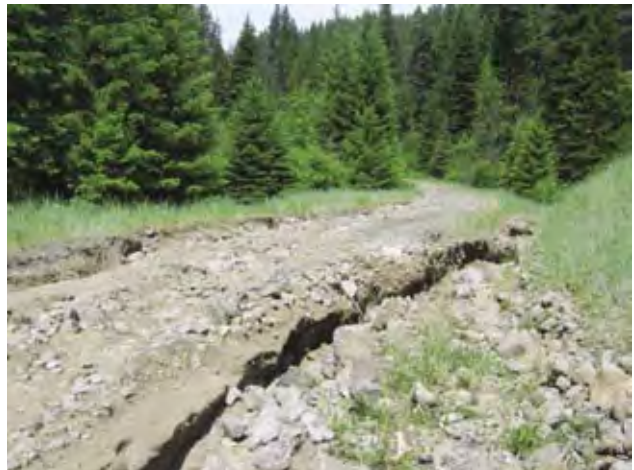
Washed out forest roads are a potentially significant source of accelerated sediment movement into wetlands. Grant County, Oregon.
