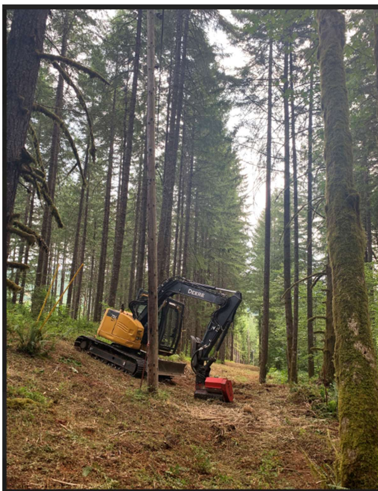
Figure 16: SlashBuster Clearing Right-of-Way
