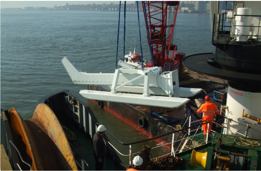
Photos of the Hudson Transmission Project (clockwise from top left): The hydro plow is lowered into New York's Hudson River prior to submarine cable burial; conduit installed under New Jersey's Bellman Creek by HDD transitions to duct bank burial; underground cable installation nears completion in a public right-of way in Fairview, New Jersey; the final phase of construction is underway at the Hudson back-to-back converter station in Ridgefield, New Jersey.
