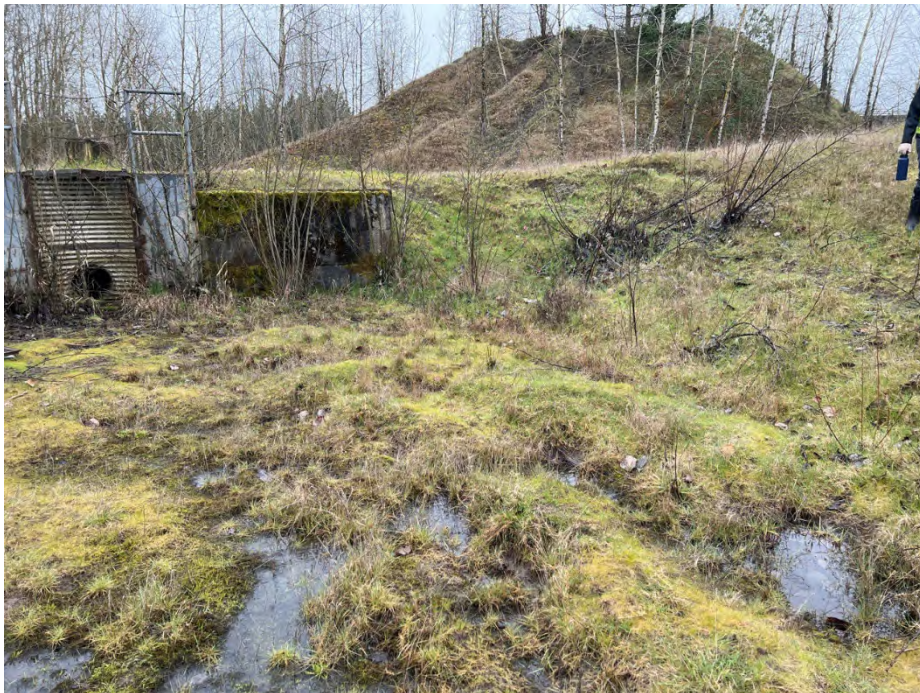
Photo 24 Sample Plot Area A-P1 (W) taken within suspect depressional area in human-made stormwater feature. Culvert discharge to 12-inch pipe to Columbia River shoreline. No evidence of flow observed. Date: 03/11/24 Direction: Southeast
