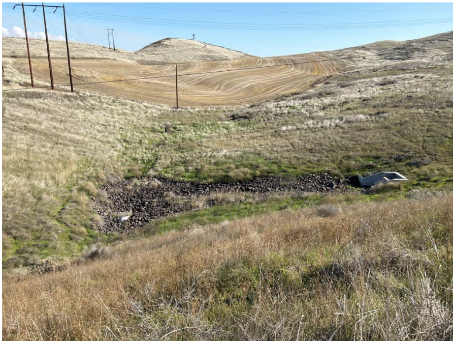
Photo 3b Looking upstream at an ephemeral drainage (Drainage 1) beneath Columbia View Drive, culvert occurs roughly 75 feet below road grade. Date: 11/08/23 Direction: Northeast
