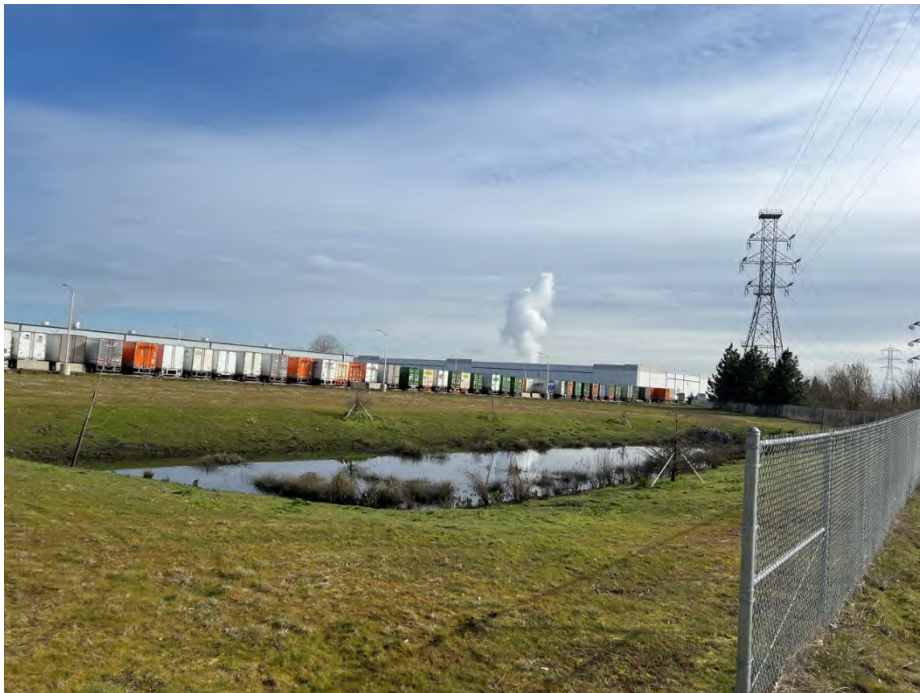
Photo 39 Stormwater feature near landing site on the east side of the Willamette River. Date: 03/13/24 Direction: Northeast
