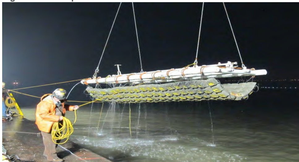
Figure 1-2. Example of Articulated Concrete Block Mat
