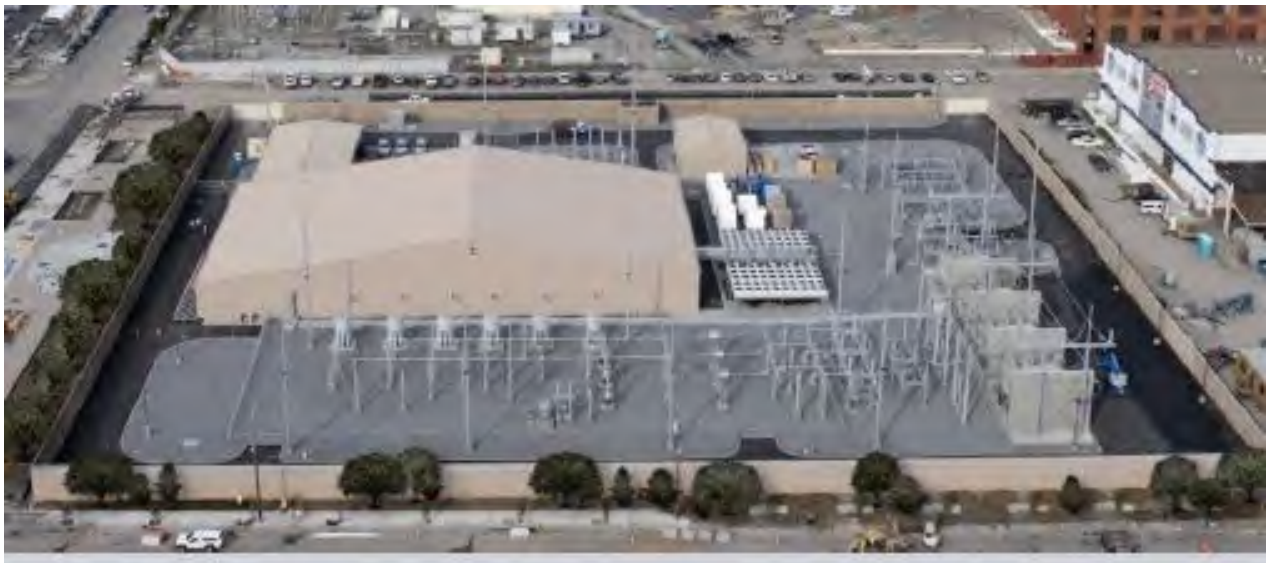
Figure 1. Typical Converter Station Layout
