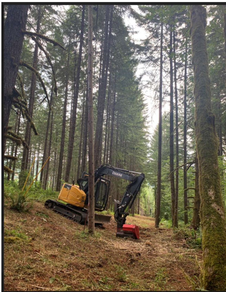
Figure 16: SlashBuster Clearing Right-of-Way
