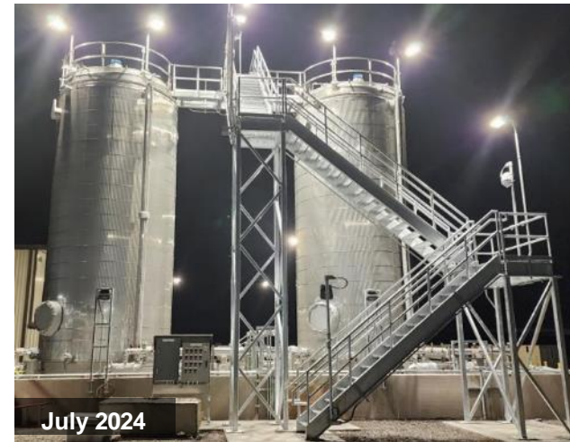
Acetonitrile distillate storage tanks
