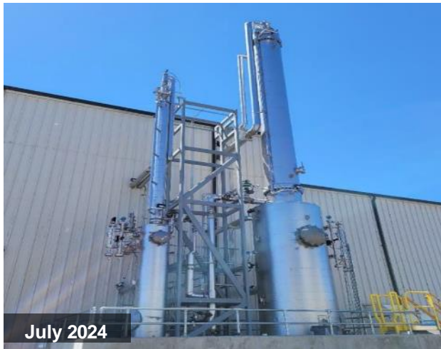
Steam stripper and concentrator columns
