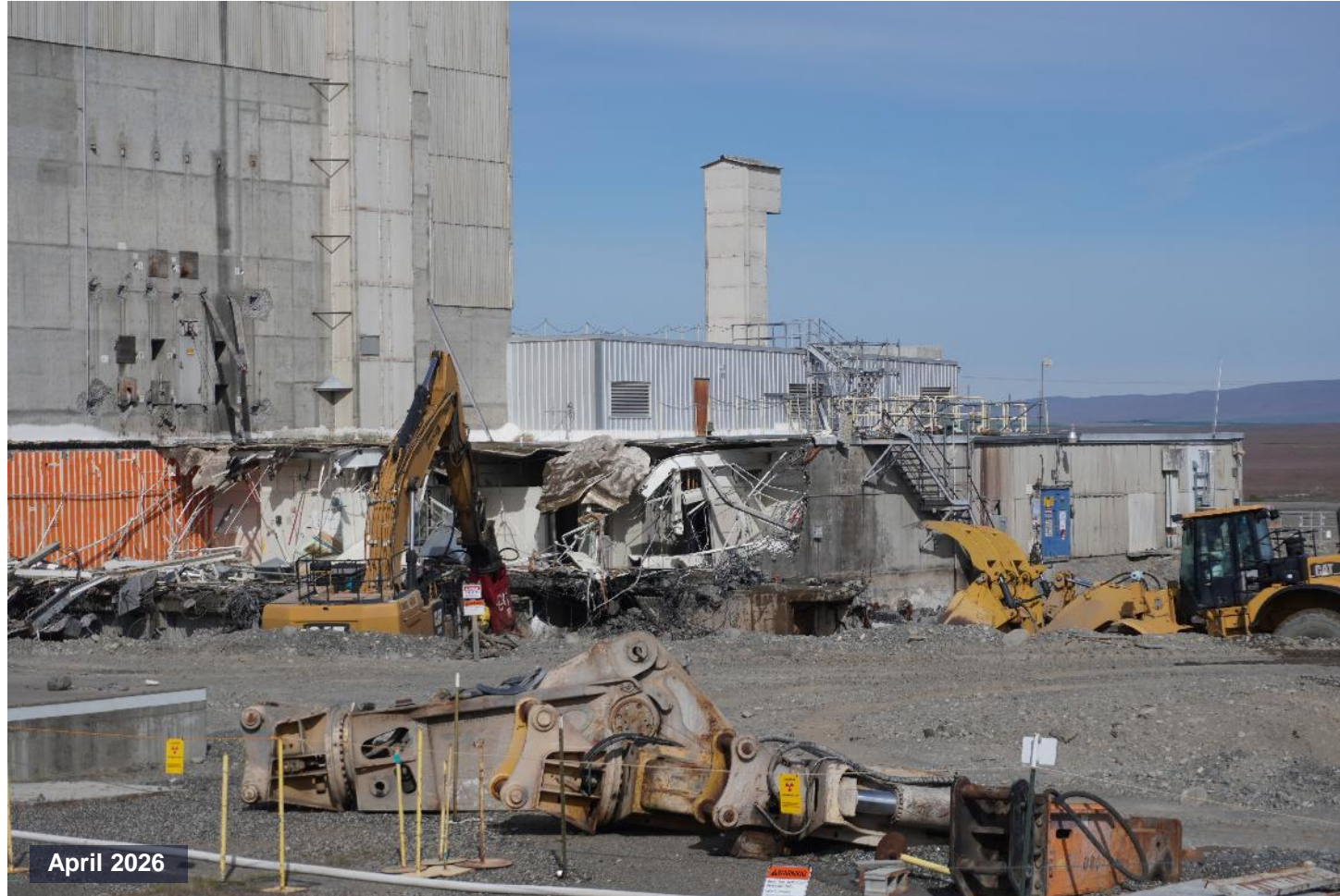
The demolition team works belowgrade to demolish the reactor's administrative areas.
