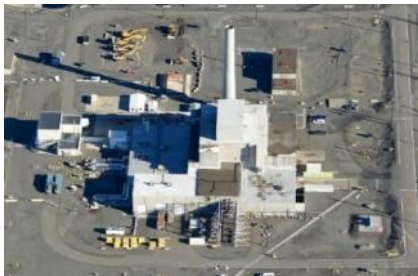
105 K West Reactor
