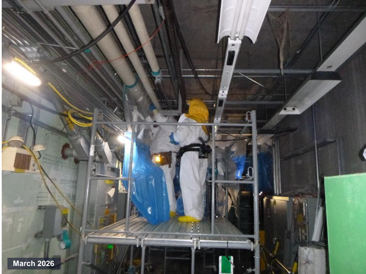
Crews remove asbestos-containing insulation from the reactor's used nuclear fuel basin.
