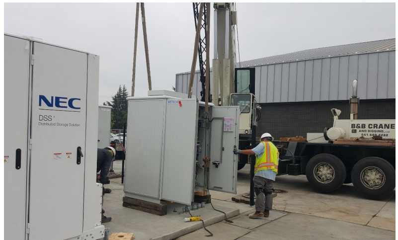
EWEB contractor installs back-up battery power system.
