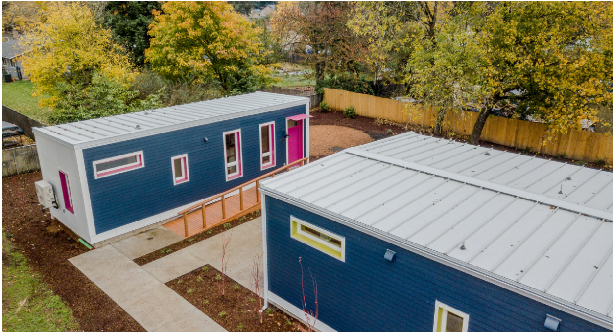
Portland Mass Casitas; Source: Adam Ramos Photography via Salazar Architect
