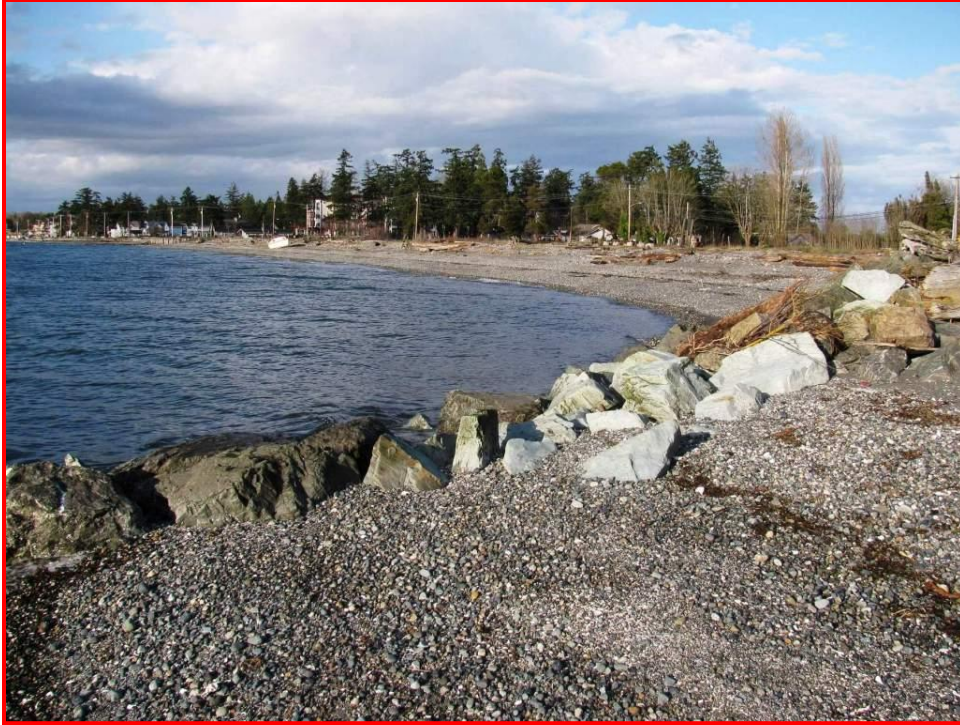
Figure 9: This riprap groin is preventing sediment from travelling along the beach. (Hugh Shipman photo.)
