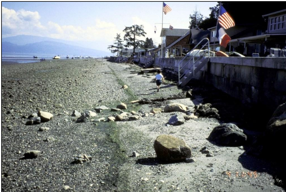
Figure 16: Samish Island, before soft stabilization.
