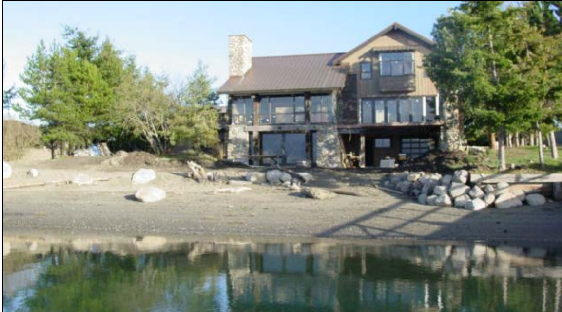
Figure 29: Fisherman’s Bay, Lopez Island after bulkhead removal and soft stabilization. (Peter Kilpatrick, Ravenhill Construction Inc. photo.)
