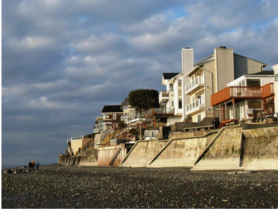
Figure 4: Single family residential community where proximity to the water and current development condition may limit soft shoreline stabilization feasibility. (Hugh Shipman photo.)
