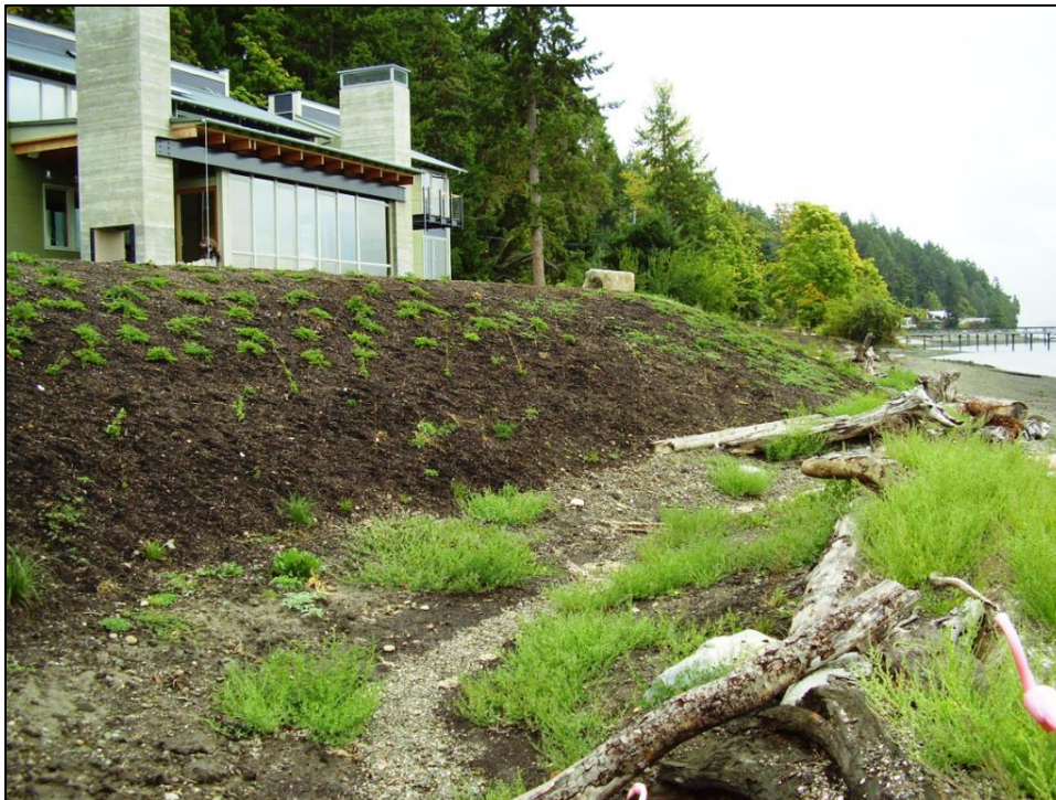
Figure 22: Port Blakely Harbor, Bainbridge Island, after stabilization.
