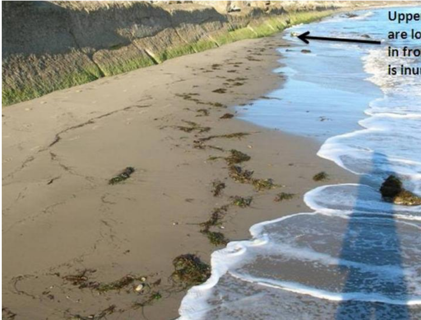
This view, looking east along an old concrete seawall on the Gaviota coast of California at low tide, illustrates the loss of ecologically important intertidal zones on a beach seaward of coastal armoring. Credit: David Hubbard
