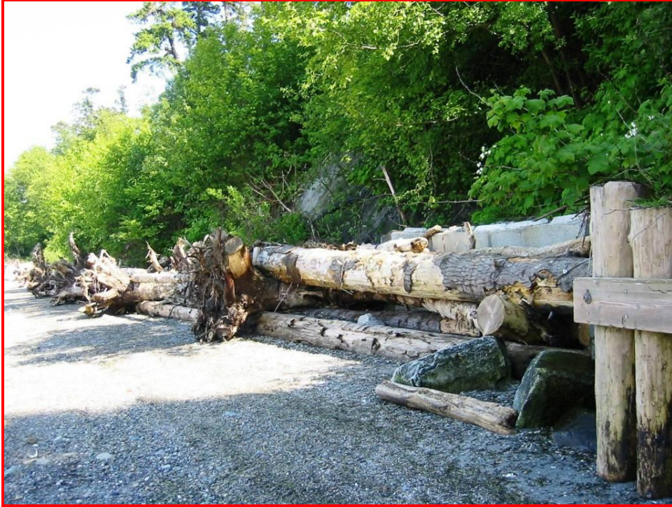
Figure 15: A log crib alternative that has many of the characteristics of a traditional bulkhead.
