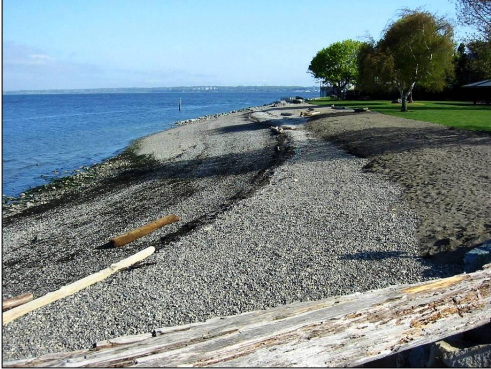
Figure 21: Marine Park, Bellingham after soft stabilization. (Hugh Shipman photo.)
