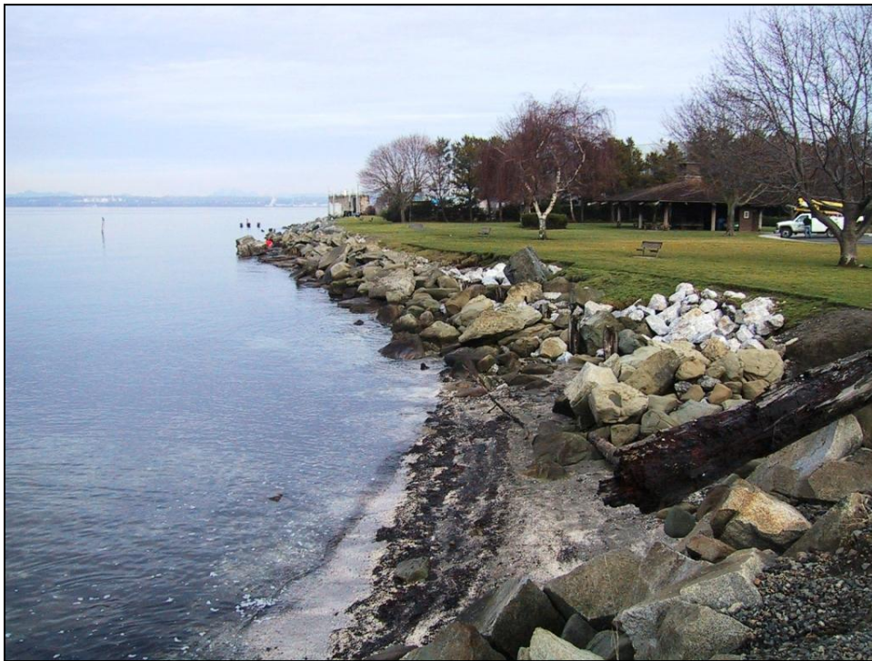
Figure 20: Marine Park, Bellingham before soft stabilization.
