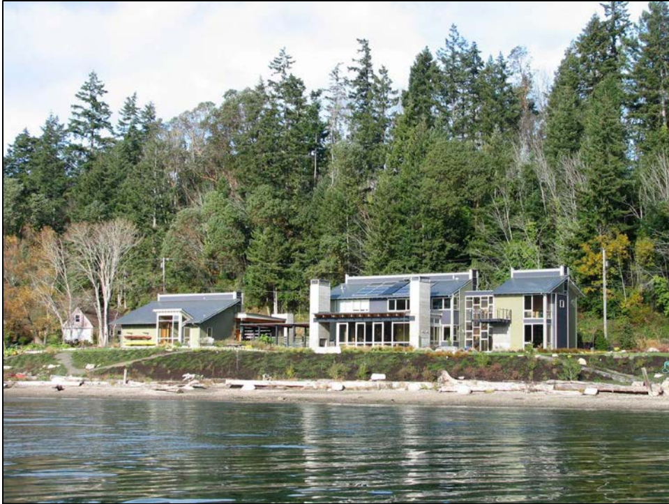
Figure 23: Port Blakely Harbor, Bainbridge after soft shoreline stabilization; view from water.
