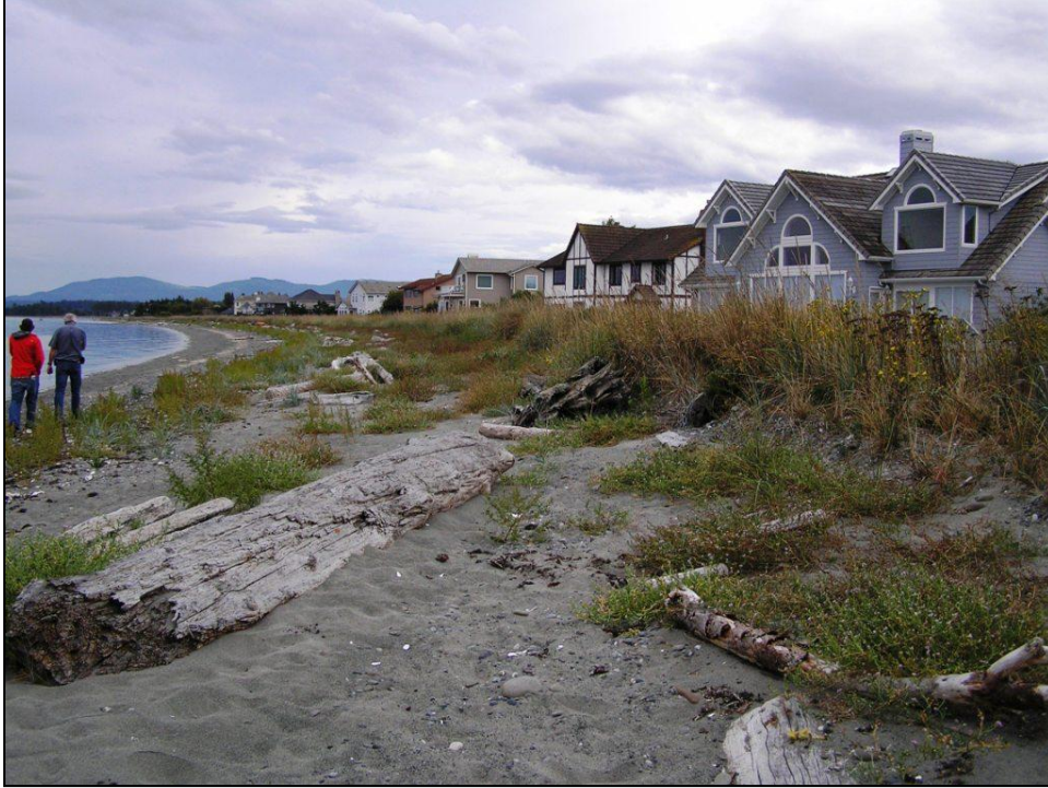
Figure 19: Seashore Lane after soft shoreline stabilization.
