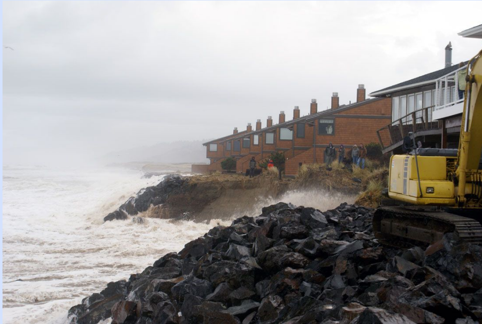
Figure 6.14. Loss of beach at Neskowin has increased the potential for waves to damage coastal structures built to protect properties as well as increased the potential for flooding of homes built behind the structures.
