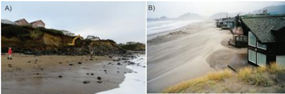
Figure 3.3.1-2: A) Emergency riprap being placed in front of a home at Gleneden Beach following a bluff failure (February 2013). B) Homes being inundated with excess sand during strong wind event in November 2021
