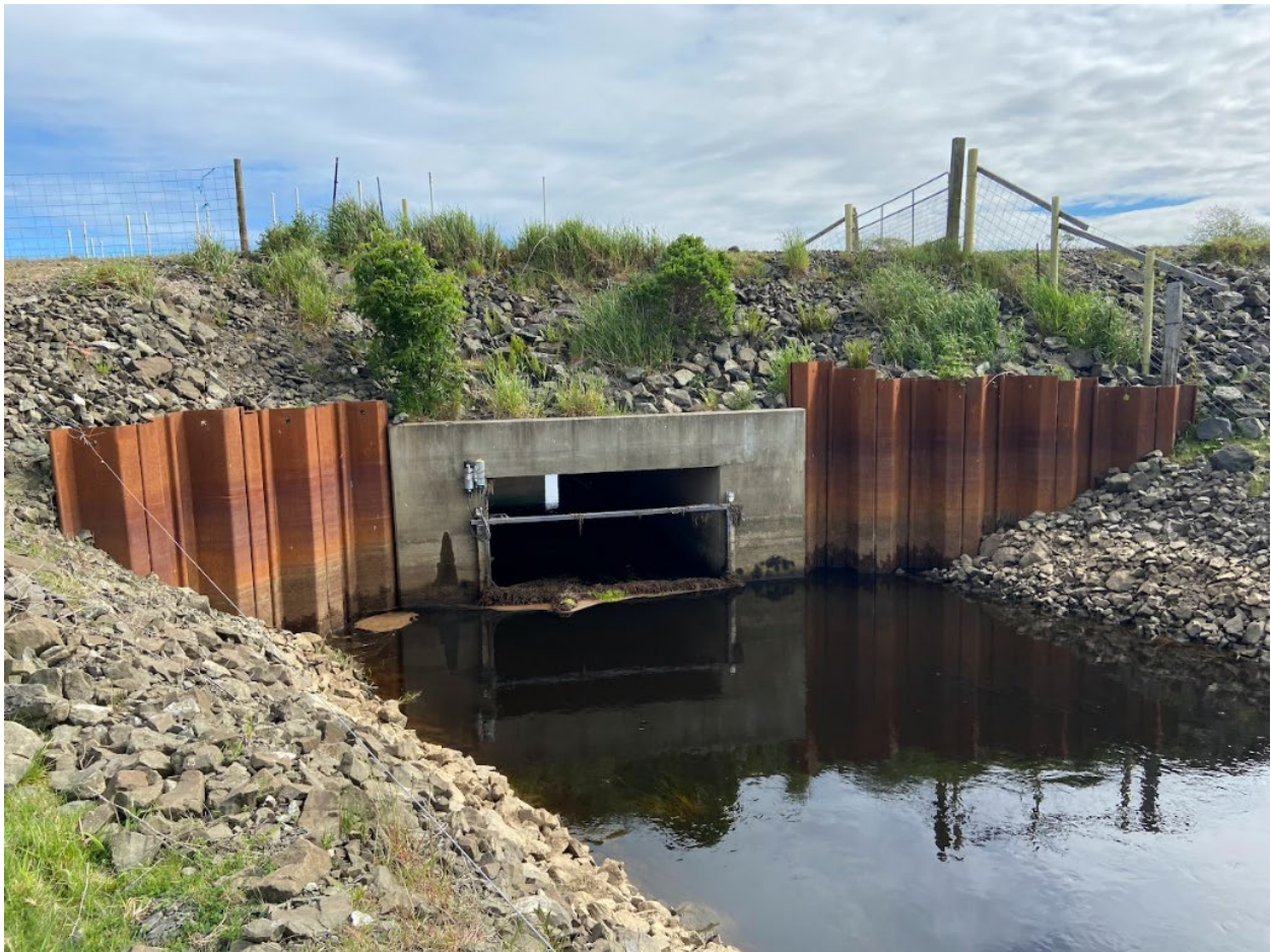
Tide gate at Winter Lake, Coquille River, 2022. Photo courtesy of Michael Moses.
