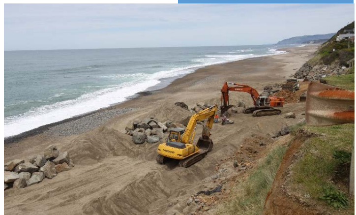
Riprap placement along Gleneden Beach in Lincoln County, 2010.
