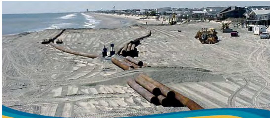
Beach nourishment, which adds sand to the coastal system, protects people and property from the effects of hurricanes and coastal storms by widening a beach and advancing the shoreline seaward. This project was constructed at Panama City Beach, Fla.
