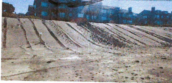
Berm restoration below residences. (Fall, 2018.)
