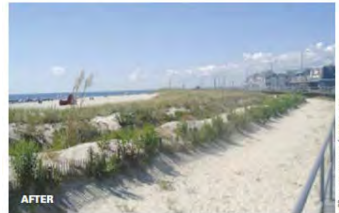
Dunes included in a beach nourishment project act as a protective barrier, preventing flooding and storm damage caused by storm surge, wave runup, and overtopping. This project was constructed at Ocean City, N.J.
