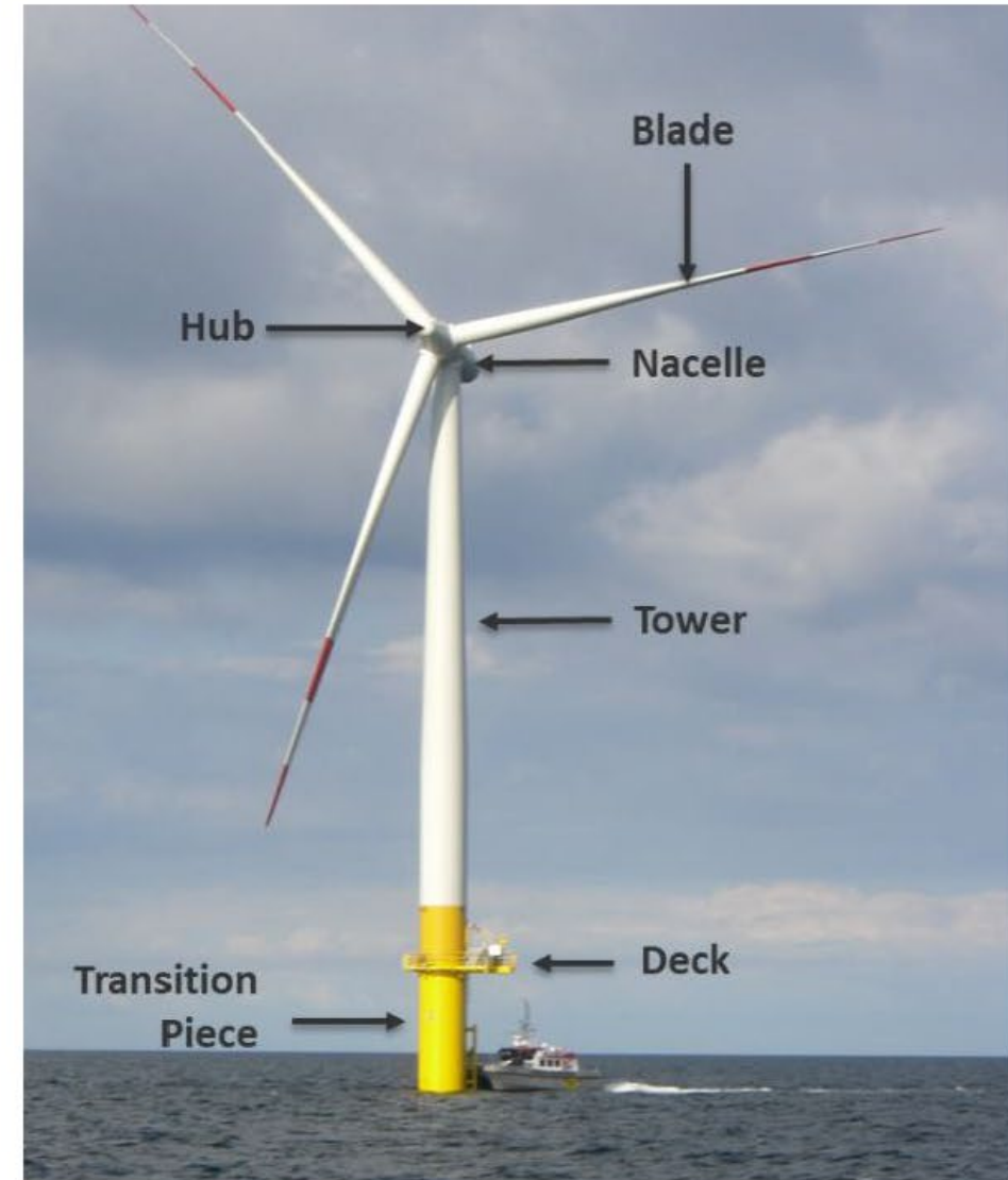
The Siemens 2.3-MW offshore wind turbine in the Baltic Sea, Germany. Photo by Walt Musial (NREL)
