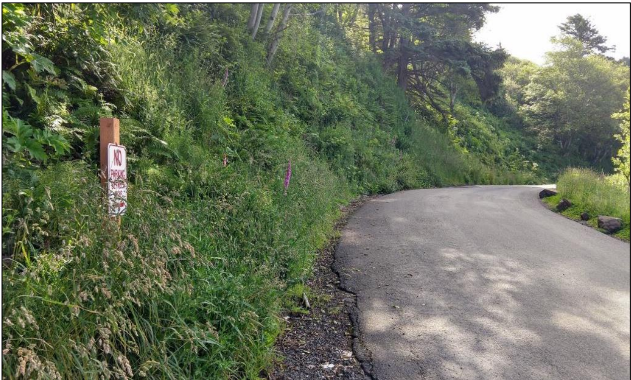
Figure 4. Location of Vault 1 along Winema Road. Vault is to be installed to frame left a short distance beyond the “No Parking” sign. View is generally east.
