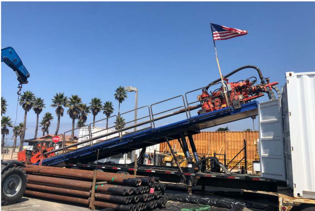
Figure 2: Example of an HDD Rig, Bore Pipes and Forklift
