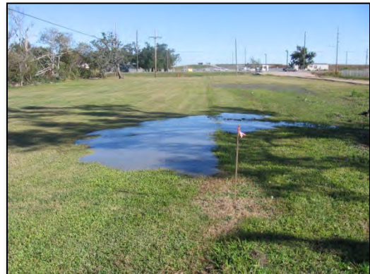
Photograph 1 - Example of Drilling Fluid Surface Release
