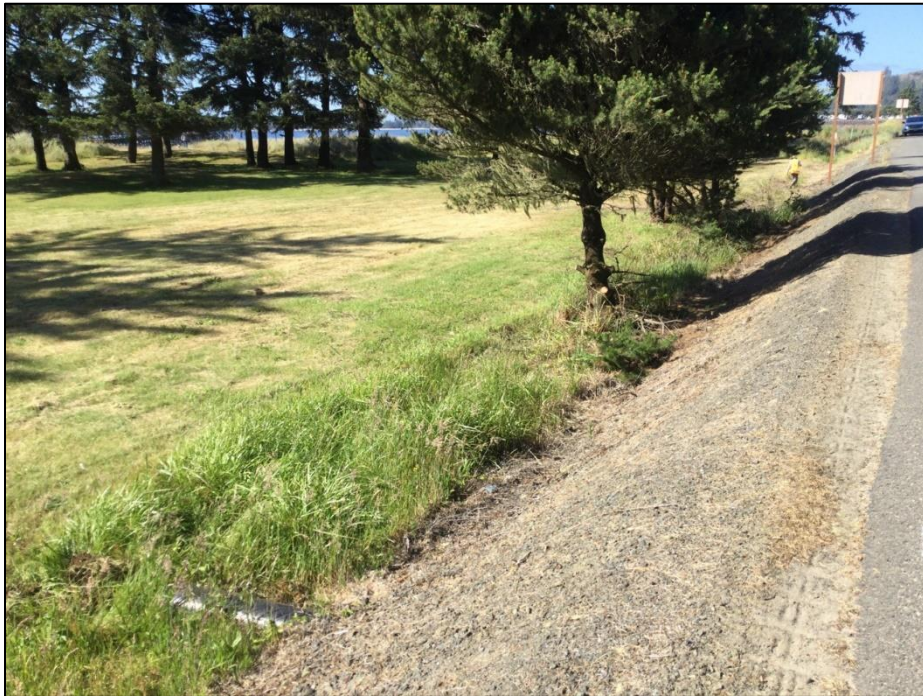
Photo 12. Ditch 1 receives water from Wetland 10 via black plastic culvert in foreground. (6/29/22)
