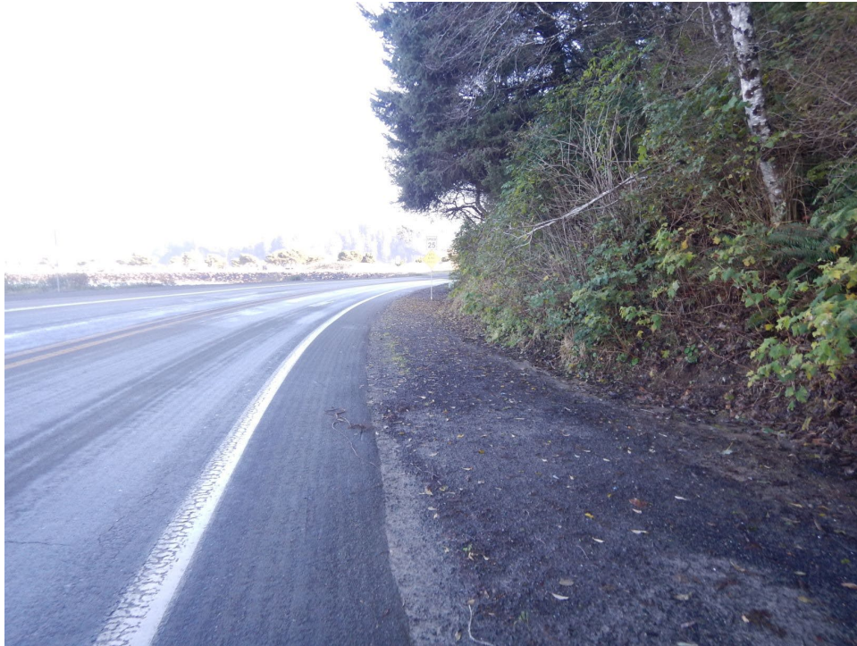
Wooded hillslope and widened paved/gravel shoulder on south side (looking Northeast)
