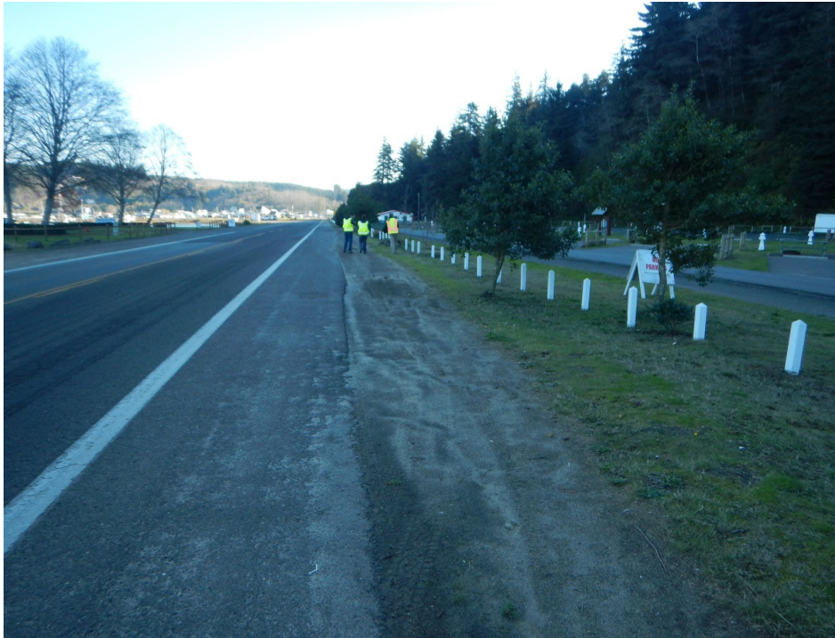
Widened paved/gravel shoulder and landscaped area south of road (looking East)
