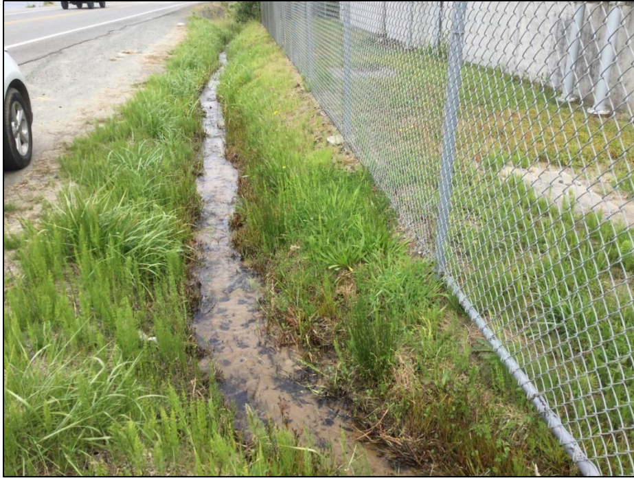
Photo 13. Stream 2 flows from bottom to top of this photo (1.5' OHW), with a narrow fringe of wetland on either side. (6/29/22)
