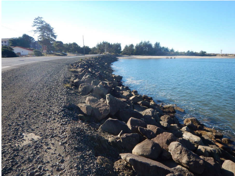
Widened gravel shoulder used by OHV directly along rocky shoreline (looking West)
