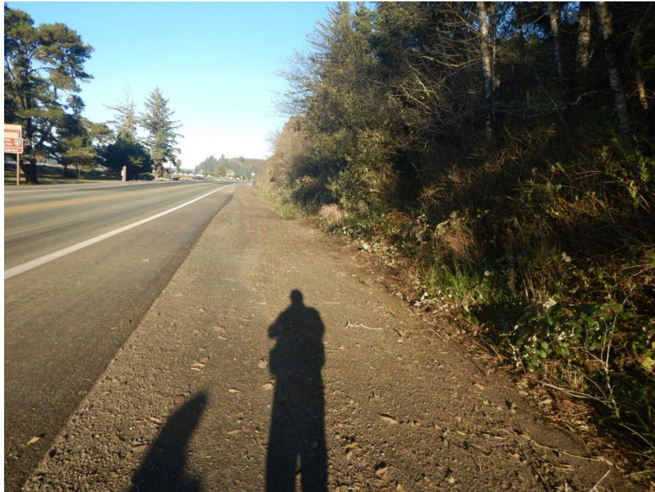
Widened paved/gravel shoulder and ditch adjacent to wooded hillside (looking Northeast)
