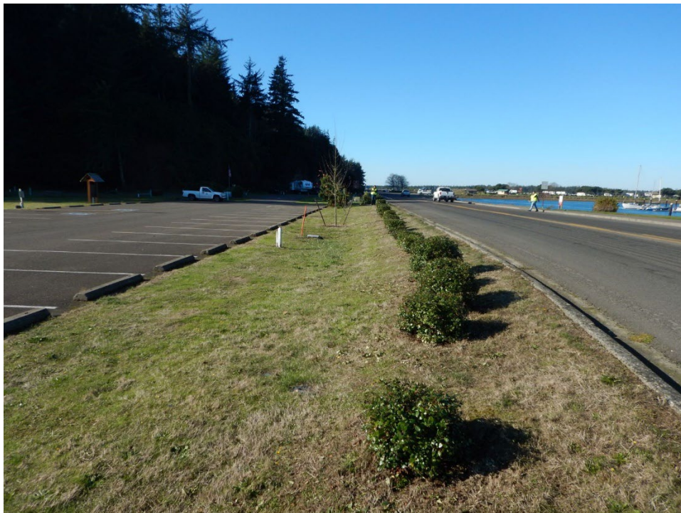
Curb & inlet storm system to be removed and landscape area south of road (looking West)
