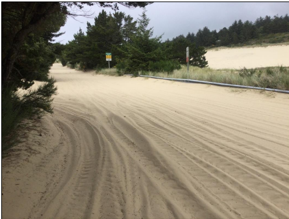
Photo 4. OHV trail looking north (6/28/22)
