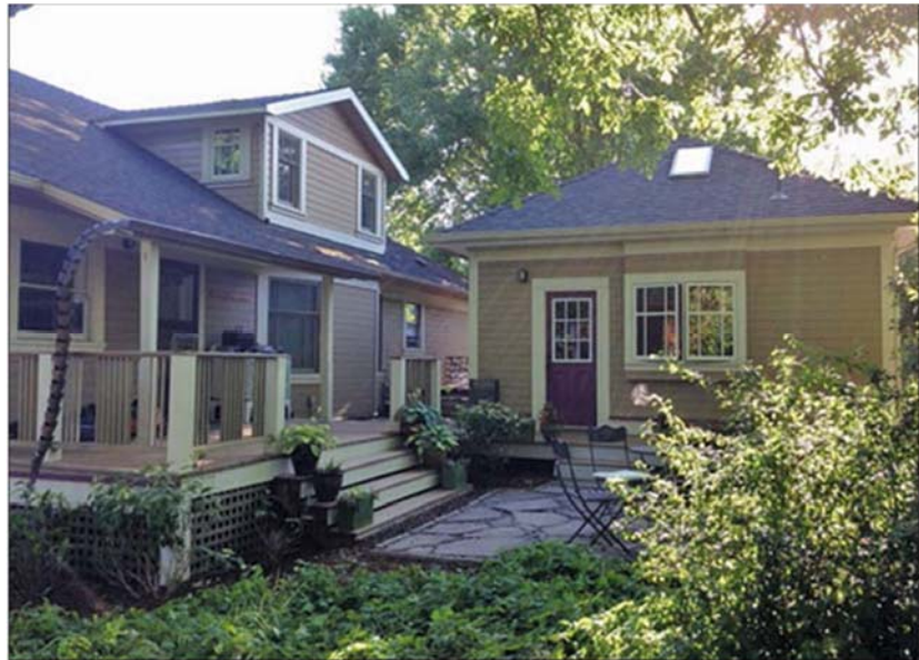
M. Klepinger's backyard detached ADU, Richmond neighborhood, Portland, OR. (Photo courtesy of Ellen Bassett and accessorydwellings.org .)
