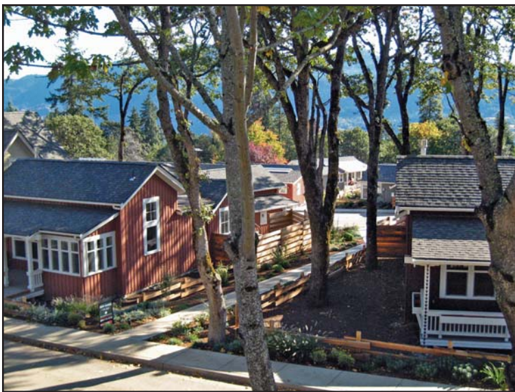
Live-work homes, Wyers End, White Salmon, WA. (Photo courtesy of Ross Chapin Architects.)
