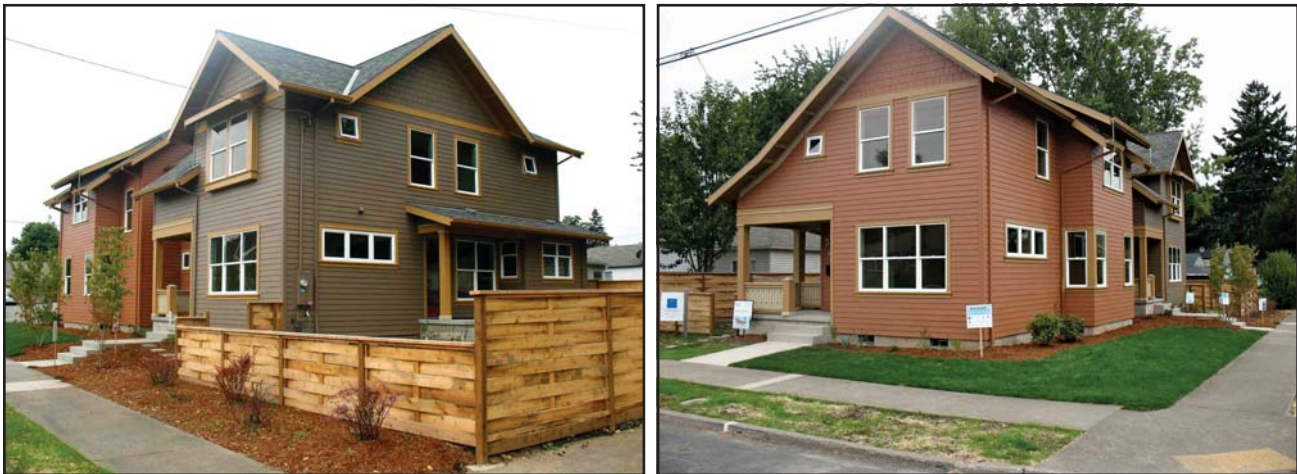
Affordable corner duplexes built by Portland Community Reinvestment Initiatives (PCRI) on N Fessenden Street, Portland, OR.
