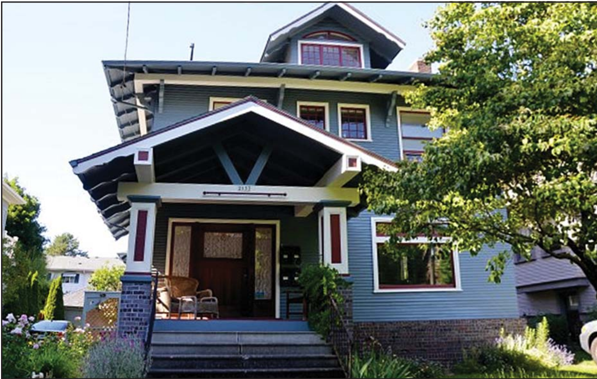
This four-plex still looks like a single-unit home from the street. (Photo courtesy of Michael Anderson, Bike Portland.)
