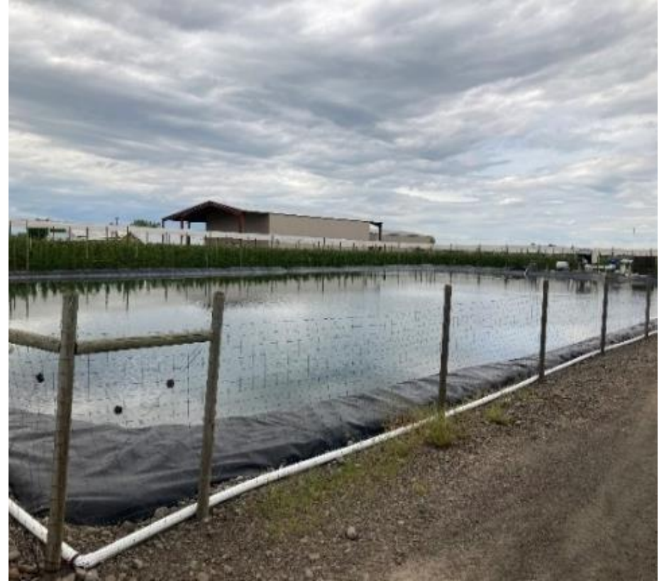
Example of a bulge in the system
