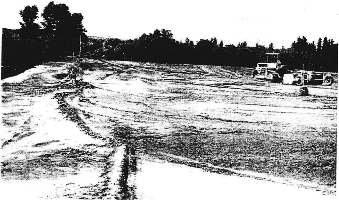
Figure 9.-Land leveling on Powval silt loam, 0 to 3 percent slopes.
