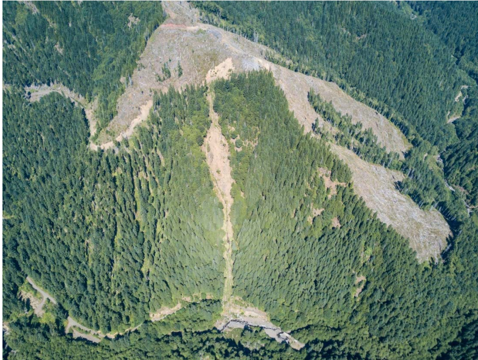
Figure 1. View of landslide triggered by the NW Combo timber sale, showing path down to West Fork of the North Fork Wilson River.
