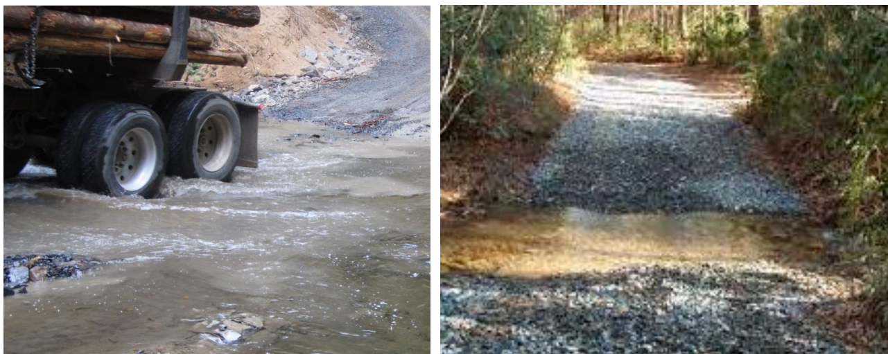
Figure 9. (left) Road is not adequately rocky and sediment is impacting the stream. (Right) Well rocked approaches with clean open rock.
