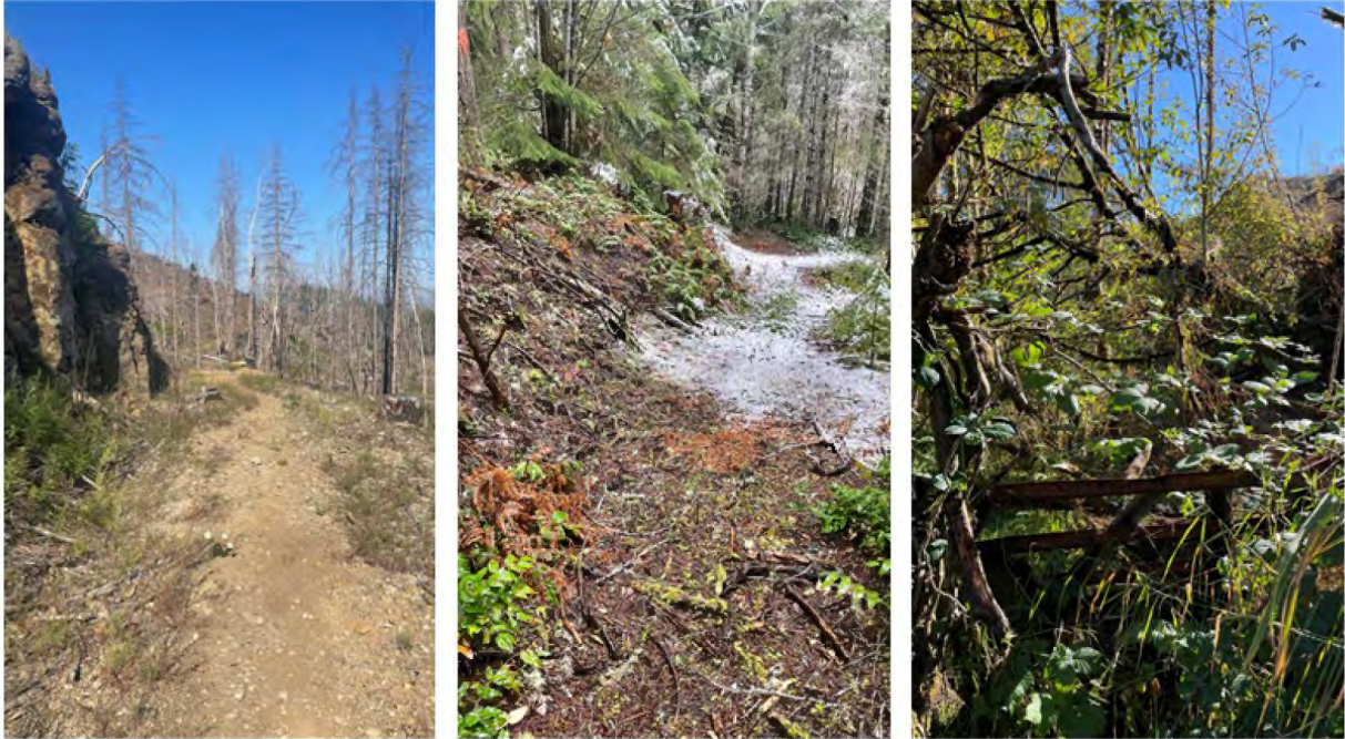
Figure 2. Examples of what an abandoned road may look like.
