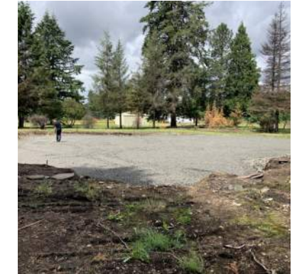
Administration building site in June, 2021
