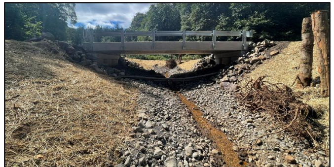
After: Clear-span bridge restoring fish passage
