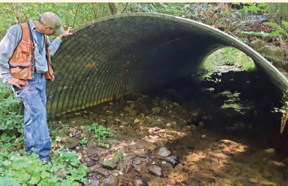
Culvert replacements like this one on Warner Creek (Astoria District) improve aquatic organism passage and restore habitat connectivity.
