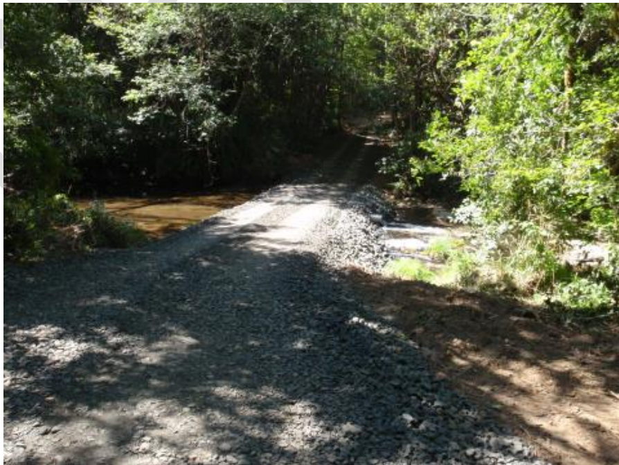
Figure 10. Temporary crossing using a culvert and rock fill.
