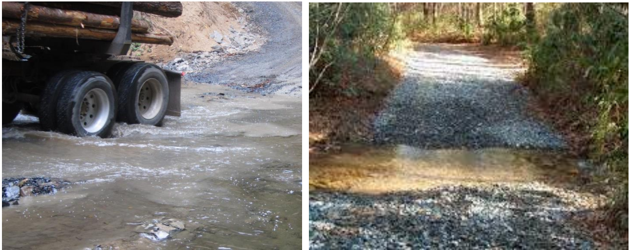
Figure 9. (left) Road is not adequately rocked and sediment is impacting the stream. (Right) Well rocked approaches with clean open rock.
