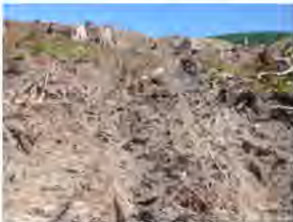
Excessive tethered equipment track depressions that are difficult to effectively drain, 10 to 24 inches deep for over 100 feet.
