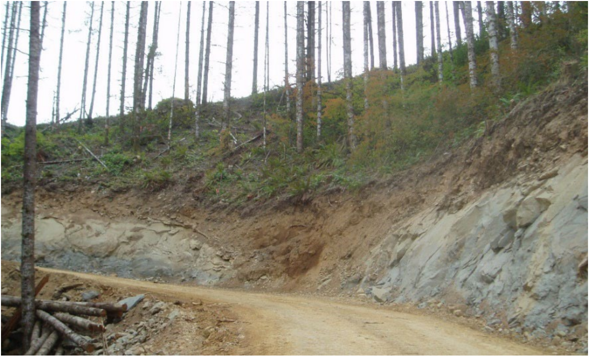
Figure I-3. Road Construction Through Headwall Depicts Deeper Soil Contained Within “U”-Shaped Bedrock
