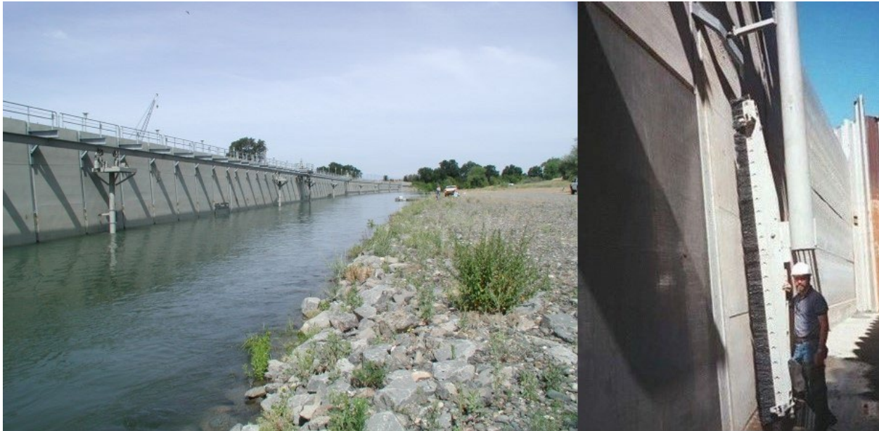
Figure 8-3 Bankline vertical flat plate fish screen sized for 3,000 ft 3 /s (Glenn-Colusa Irrigation District) along the Sacramento River in California (Note: the screen is shown in operation (left) and during construction (right).)
