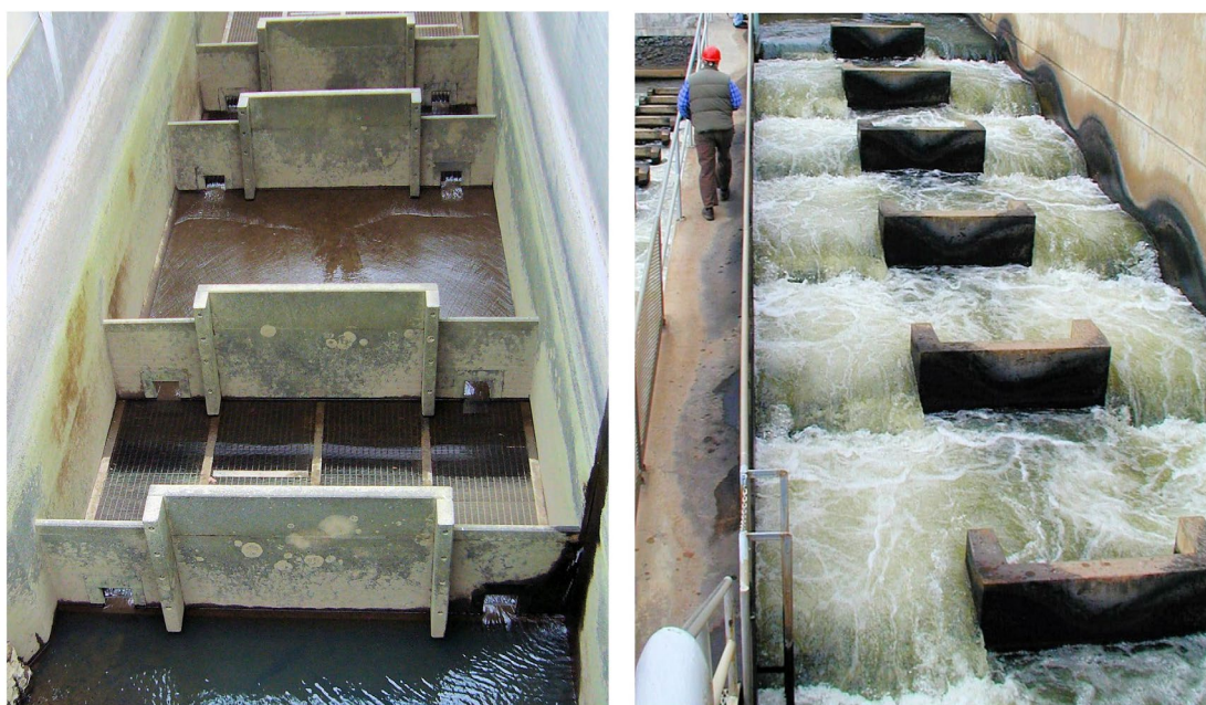
(a) Looking downstream
