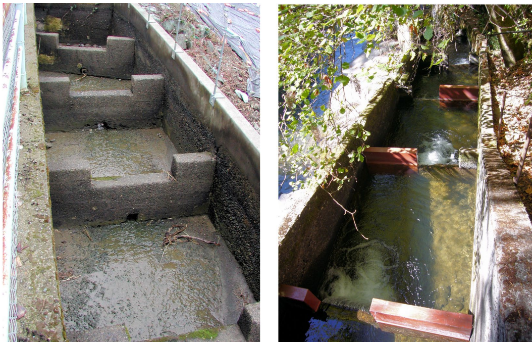
Figure 5-6. Examples of pool and weir ladders
