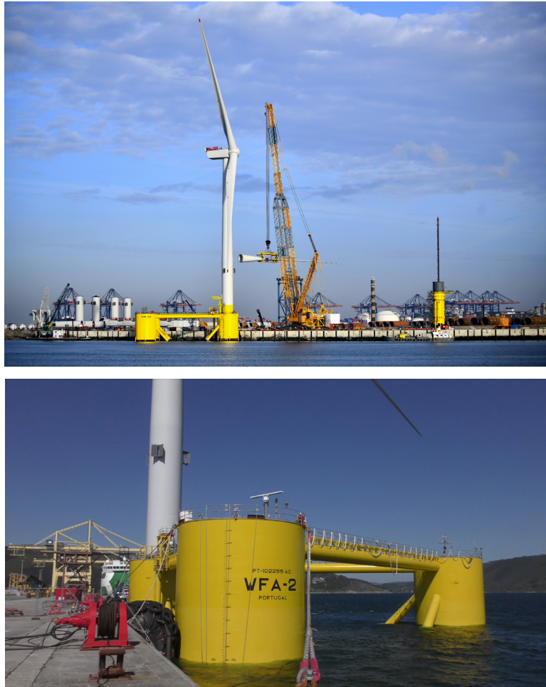
Figure 10. Floating offshore wind turbines at assembly ports. Top: Floating wind turbine (9.5 MW) for Scotland’s Kincardine Offshore Wind project at a port in The Netherlands. Bottom: Floating platform for an 8.4 MW Floating wind turbine for Portugal’s WindFloat Atlantic project along a quay in Spain (for scale, note the figure in red coveralls at the top right side of the floating platform). Photographs courtesy of Principle Power.
