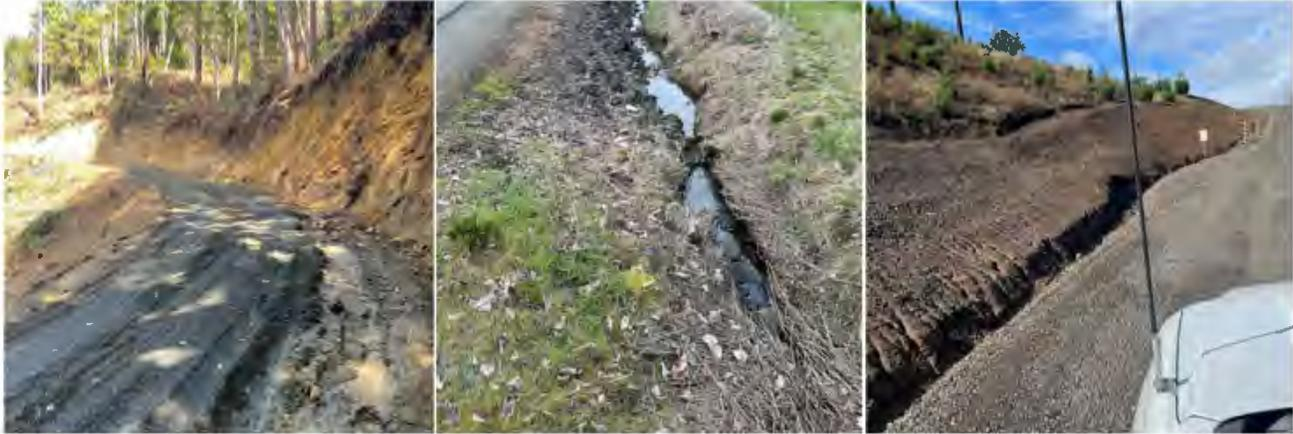
The road has sinkholes. (Not a pothole, but a hole that can't be driven over.)
