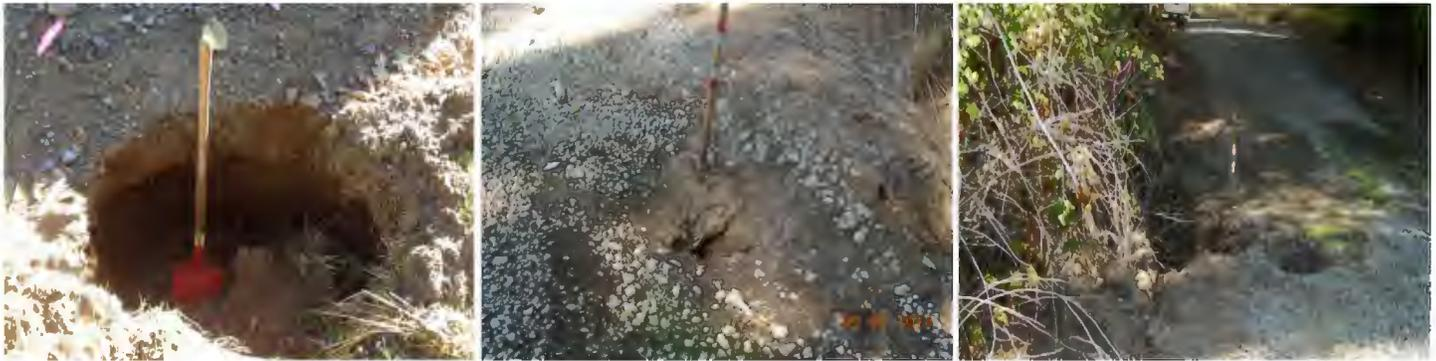
Dirt from the uphill side of the road is moving towards or falling into the road ditch or has signs of erosion.
