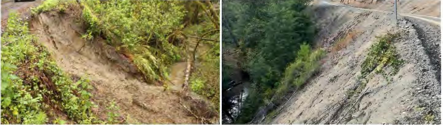
There are cracks on the outside edge of the road, road fill is on top of vegetation or debris, or there are nearby landslides.
