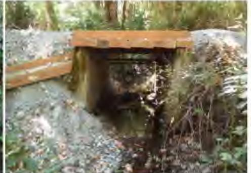
Streambed material does not cover the bottom of the culvert throughout its entire length on the inside.
