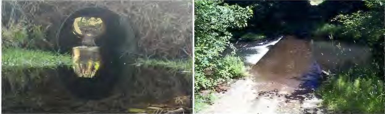
The water depth across the ford or in the culvert is shallower than in the adjacent stream channel.
