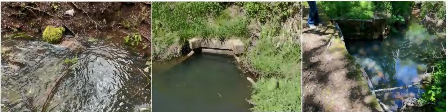
The culvert is clogged or keeps clogging with dirt or debris.
