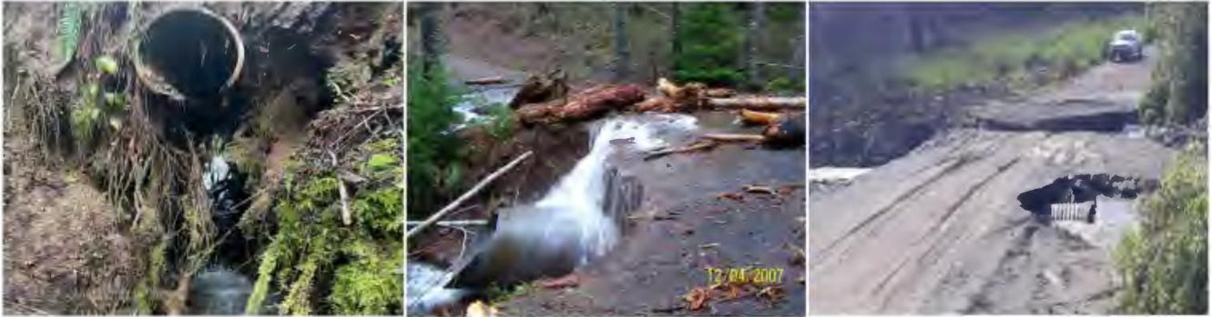
There is ponding of water upstream of the culvert.
