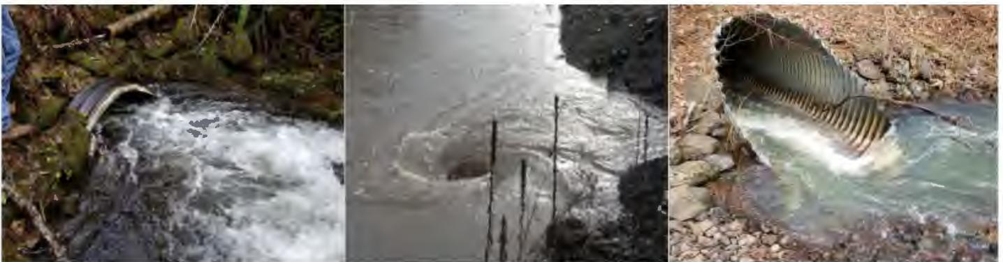
Dirt from the fill over the culvert is falling into the stream.
