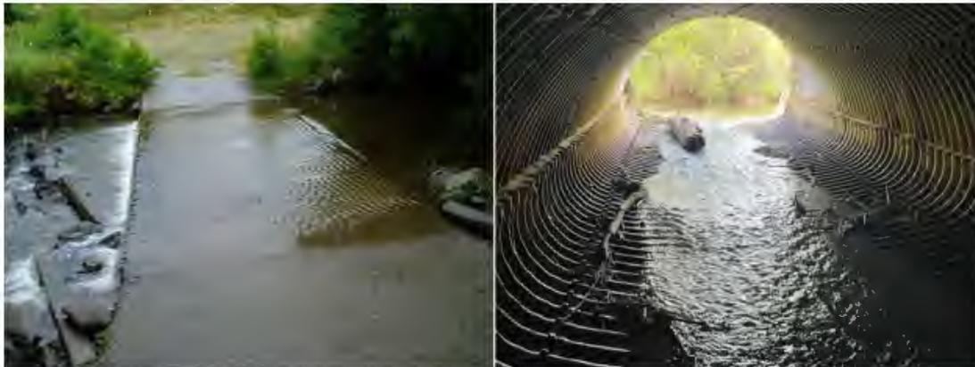
Fish have difficulty swimming through or over the water crossing because of fast moving water.
