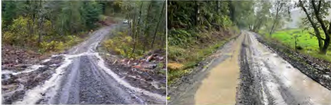
There are signs of erosion or sediment present on the road surface.
