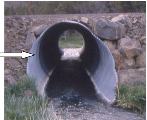
B. Non-perched culvert. Note that the culvert is embedded so the stream flows through without a major change in streambed elevation.
