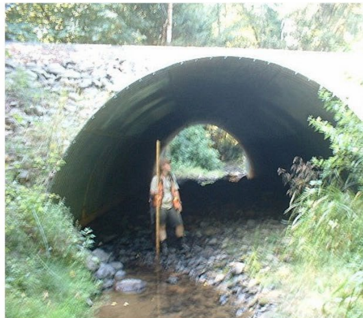
C. Open-bottom arch culvert.
