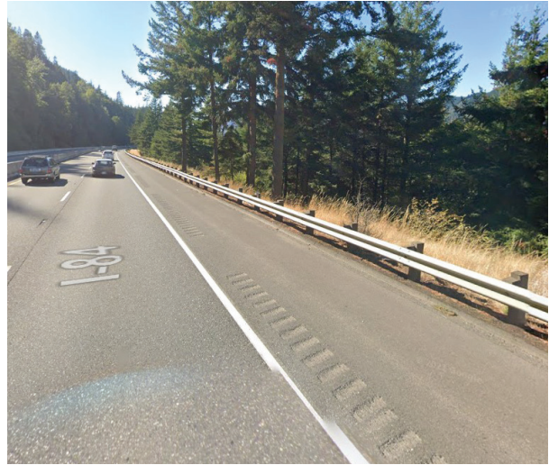
Existing shoulder on I-84 westbound
