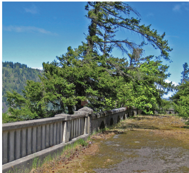
Section of historic road and masonry railing at Ruthton Point
