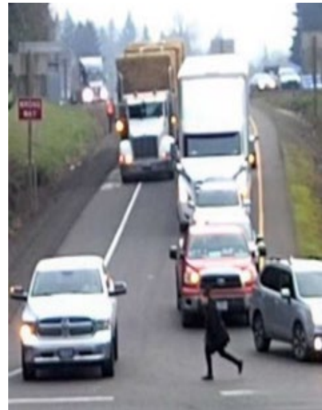
Pedestrian crossing at stop-controlled ramp with no pedestrian facilities.
