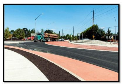
roundabout could provide adequate capacity and minimize delay under 2040 traffic conditions, accommodate freight movements, and accommodate bicycle and pedestrian users with significant safety benefits as compared to other alternatives. As a result of the RSA and the ICE, ODOT moved forward with constructing a roundabout at the Intersection to achieve safe and efficient operations of the highway.
