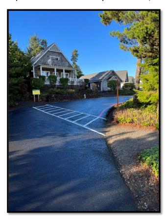
resurfaced roads, sealed cracks, and strategically placed replacement asphalt in two high-traffic zones. Perhaps most importantly, our roads are now adorned with clear and highly visible markings, including fire lanes, crosswalks, and speed bumps. This enhanced visibility contributes significantly to the safety of our residents, particularly during nighttime hours."
