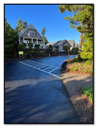
resurfaced roads, sealed cracks, and strategically placed replacement asphalt in two high-traffic zones. Perhaps most importantly, our roads are now adorned with clear and highly visible markings, including fire lanes, crosswalks, and speed bumps. This enhanced visibility contributes significantly to the safety of our residents, particularly during nighttime hours."
