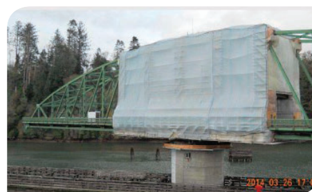
Umpqua River (Reedsport) Bridge cathodic protection.
