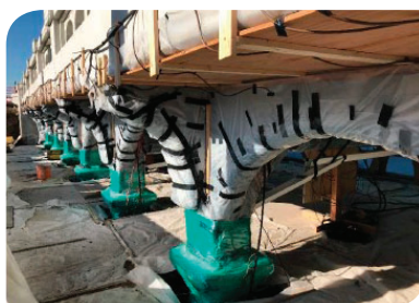
Dry Canyon Bridge (Historic Columbia River Highway) re-alkalization project.
