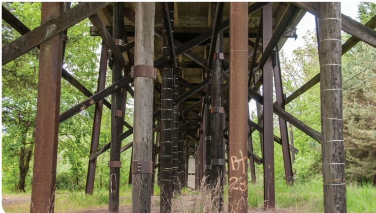
Bridge substructure with a mix of older timber and newer steel piles.
