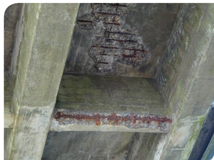
Yaquina Bay Bridge Span 4 Corrosion Damage
