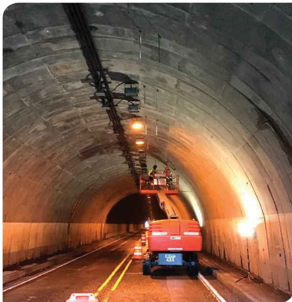
Installation of new lighting
