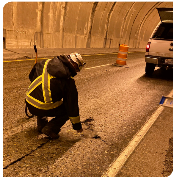
Cracking, patched spalls.
