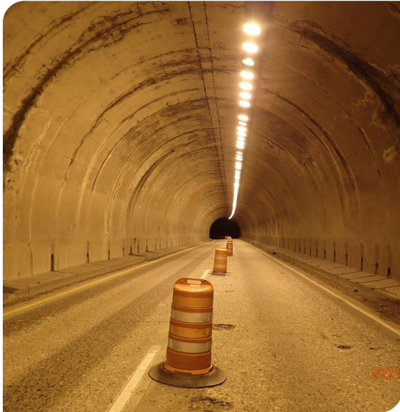
Spalling in tunnel floor.
