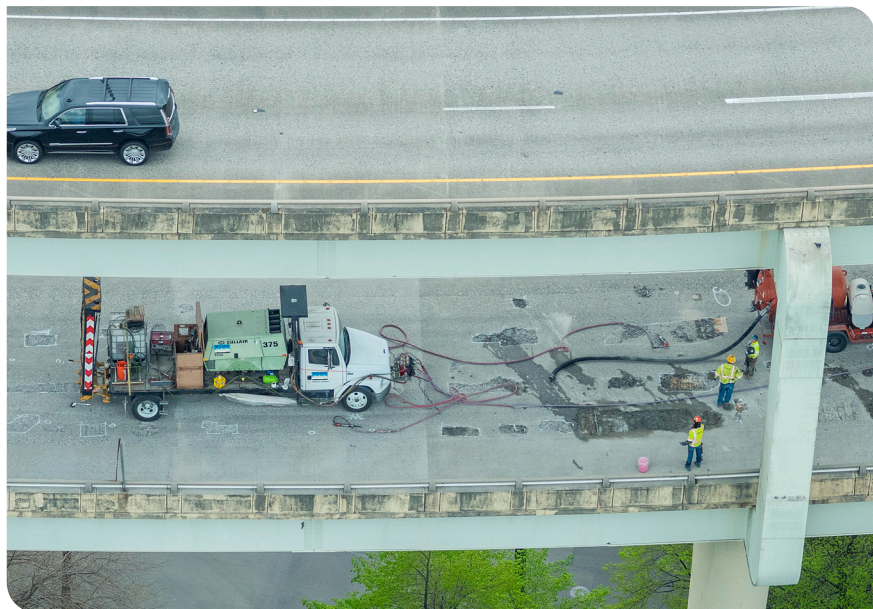
Repairing holes through the lower deck of the Fremont Bridge. This bridge was built in 1973.
