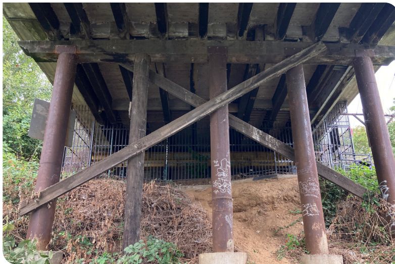
Bridge substructure with a mix of older timber and newer steel piles.
