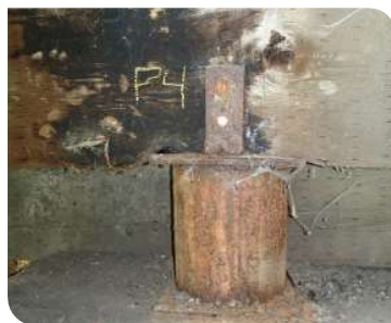
Crushed timber cap.
