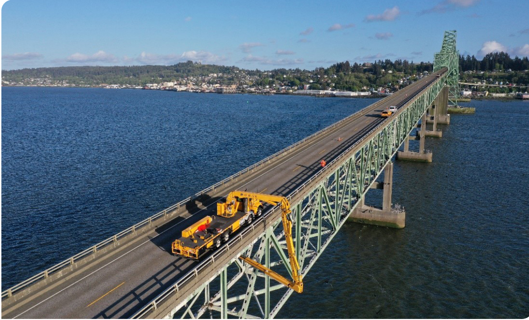
ODOT inspects the paint on the Astoria Megler bridge to prepare for an upcoming project.
