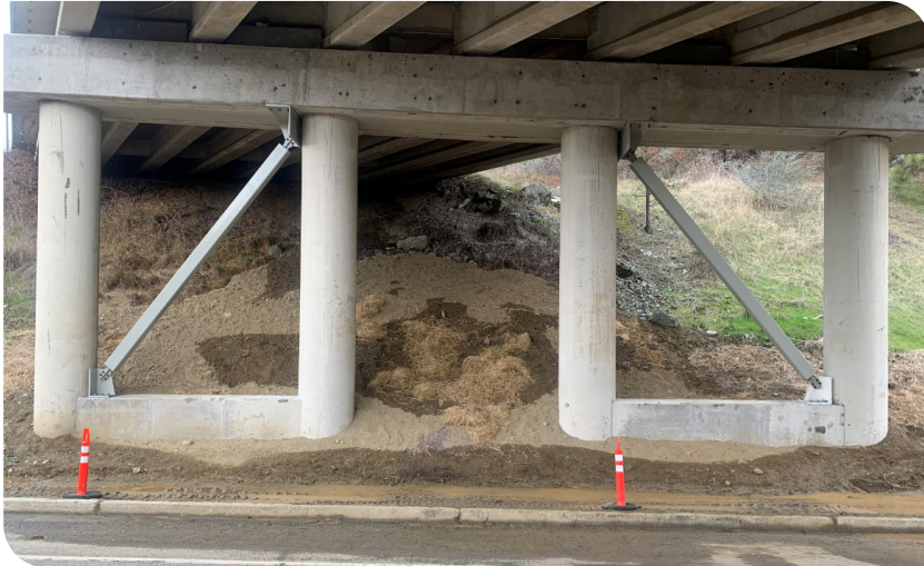
Leland Road Bridge retrofitted with buckling restraint bracing.
