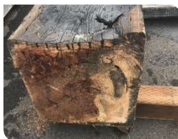
Cross section of deteriorated timber cap.
