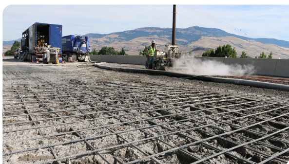
Partial depth hydro-demolition of a bridge deck.
