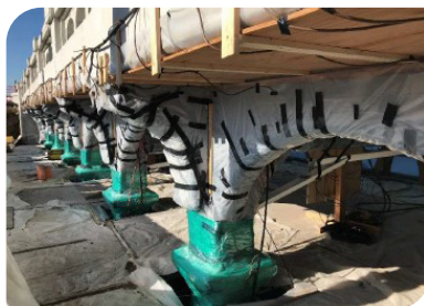
Dry Canyon Bridge (Historic Columbia River Highway) re-alkalization project.
