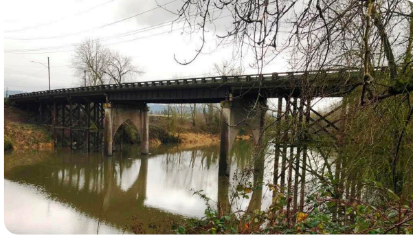
A side view of the Columbia Slough Bridge, showing the extensive use of timber for support.
