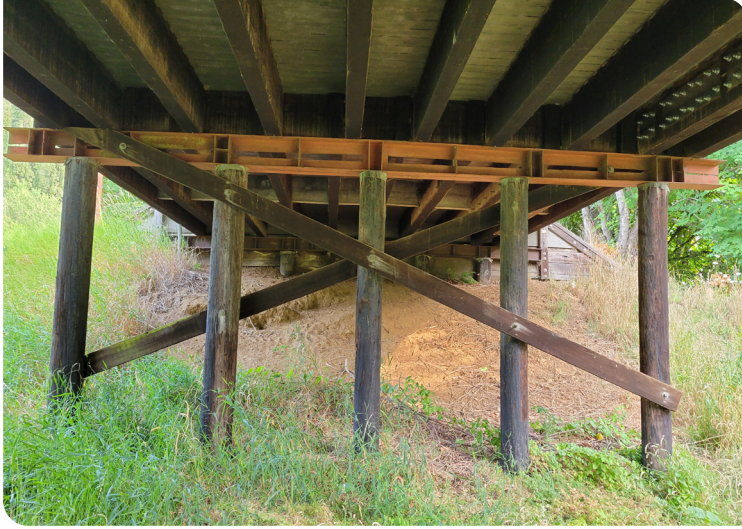
Bridge substructure with a mix of older timber and newer steel piles.
