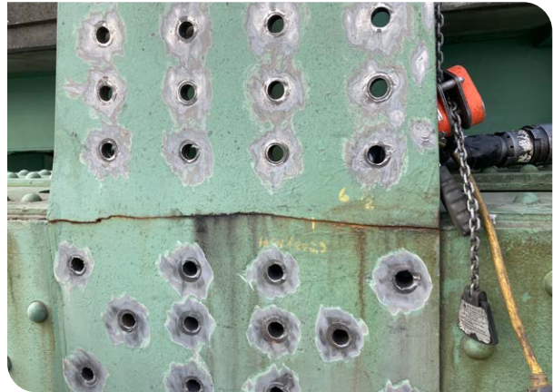
Steel Fatigue Crack
