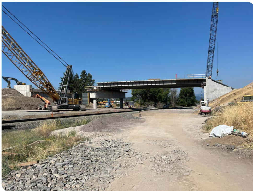
Pelican City Bridge— Placing precast concrete girders.
