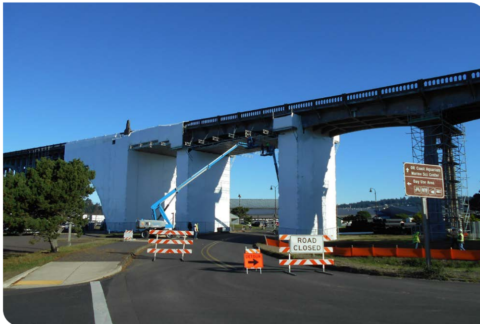
Temporary work access and containment on the Yaquina Bay Bridge (Newport, OR) – Cathodic Protection Work (2023).
