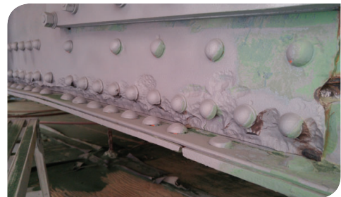
Failed paint on steel member.
