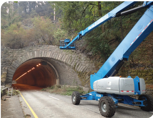
Tooth Rock Tunnel being inspected following the 2017 Eagle Creek Fire
