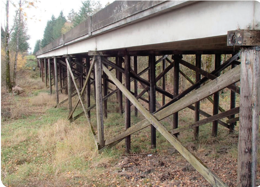
Yamhill River Overflow Bridge Timber Substructure
