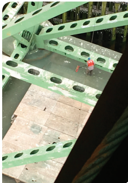
Painting preparation on the Astoria Megler Bridge.
