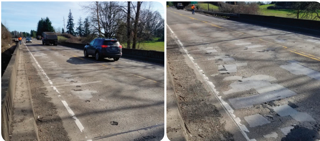
Yamhill River Overflow Bridge Deck and Patching
