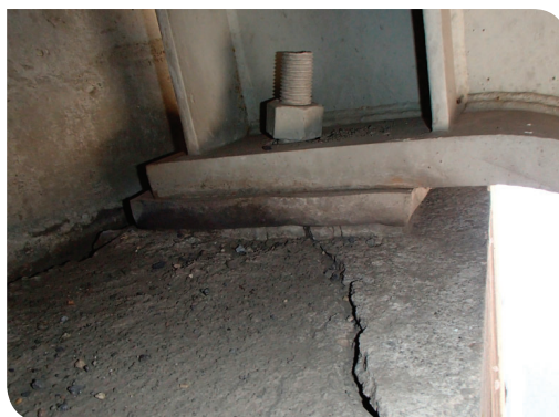
Bearing Ledge Failure
