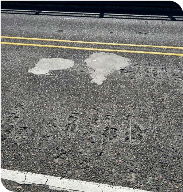
Looking northeast at the deck surface.
