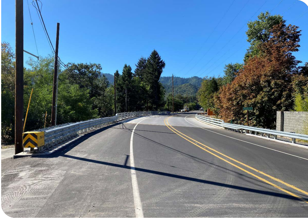
The new Foothills Creek Bridge – In addition to replacing an old deficient structure, it improved traffic safety.
