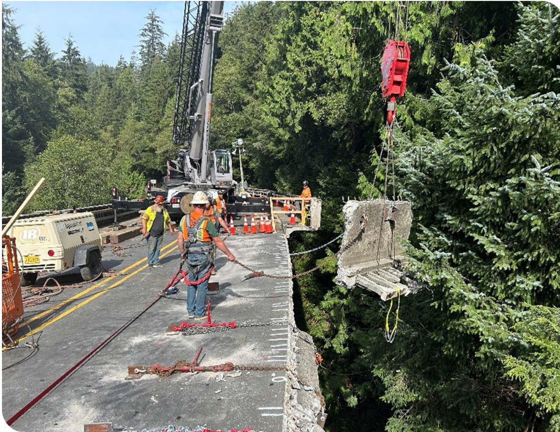
Necarney Creek Bridge, U.S. 101.
