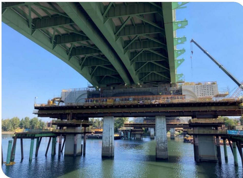
Abernethy Bridge - Construction of the crossbeams is nearing completion.
