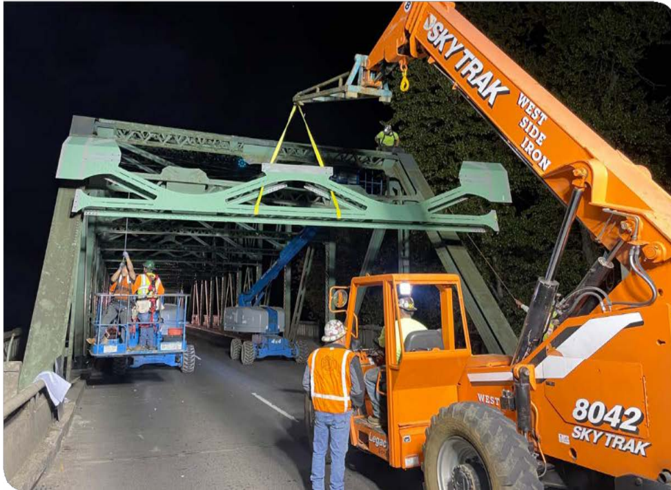
Ellsworth Bridge over the Willamette River – Portal bracing replacement (2024).
