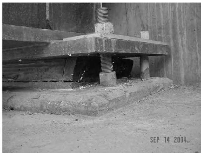
Elastomeric Pad Shift Due to Deck Deadload
