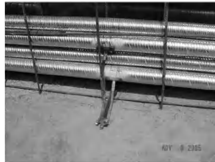
Larger stirrup spacing @ midspan
