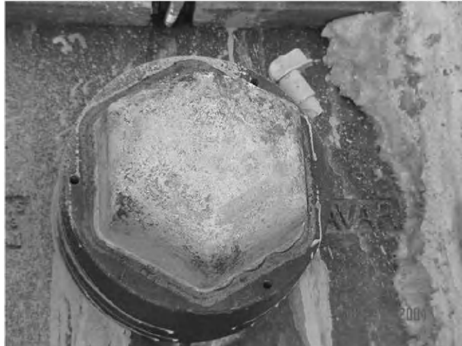
Grouted End After Cover Removed
