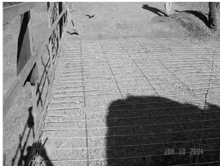
Wire Placed on Compacted Level Surface
