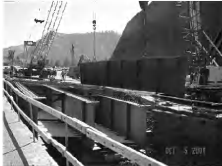
Steel Plate Girder
