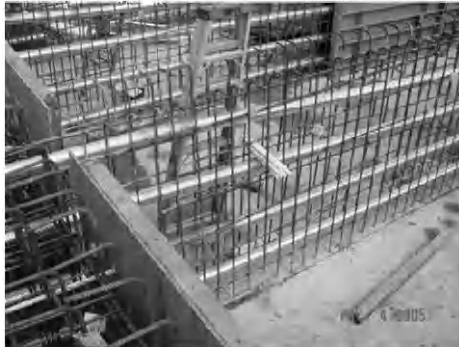
Tighter stirrup spacing near abutments
