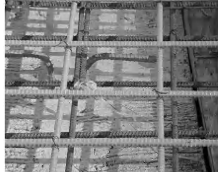
Epoxy coated ties for epoxy rebar
