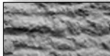
CSP 9 (heavy scarification)
