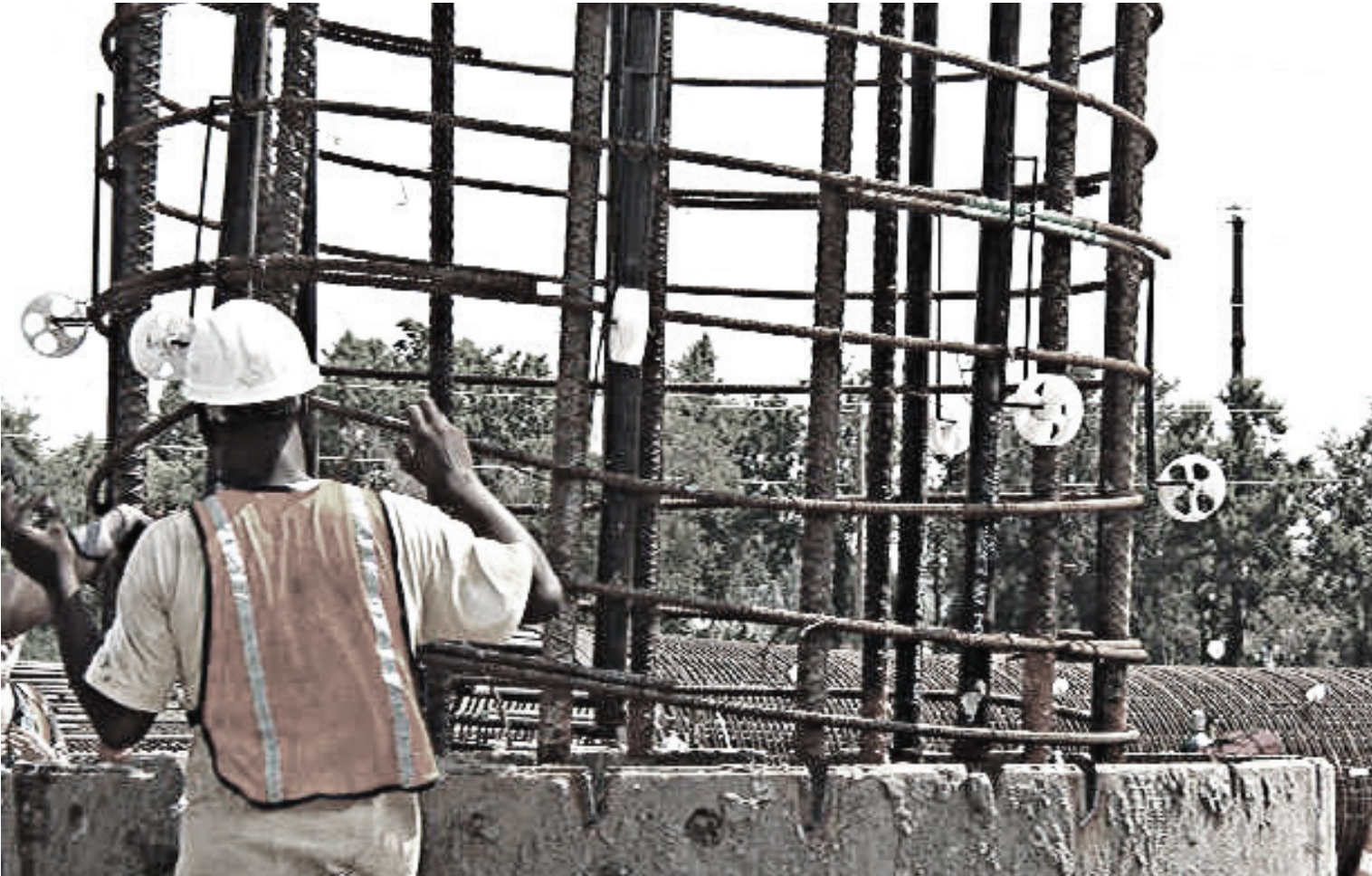
Guiding rebar cage into drilled shaft with Hairpin and ShaftSpacer system attached
