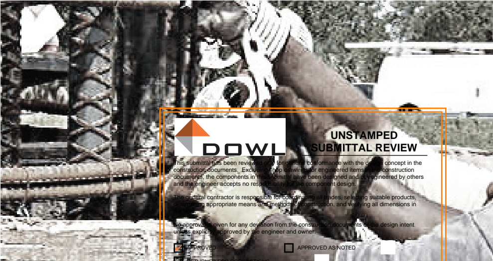
Attaching the Hairpin with tie-wire
