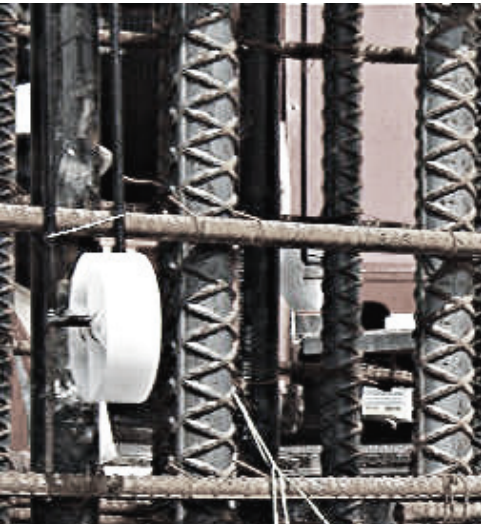
Hairpin attached to rebar cage
